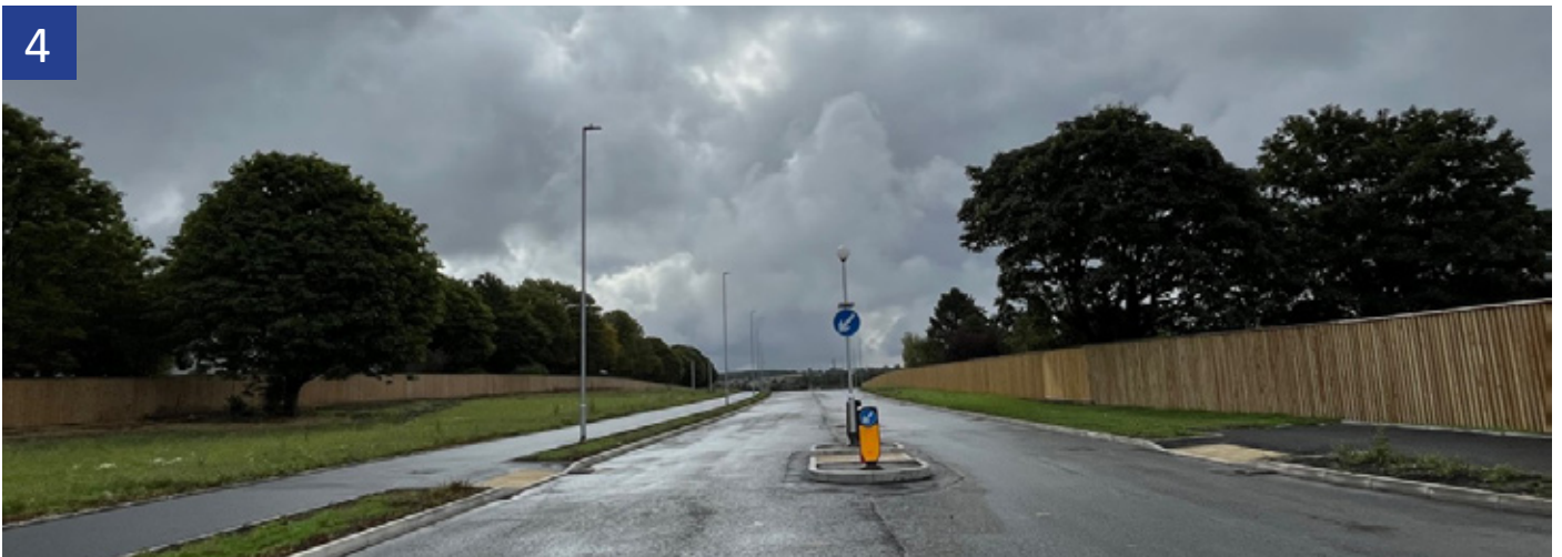
View looking north west along the new link road adjacent to the proposal site.
