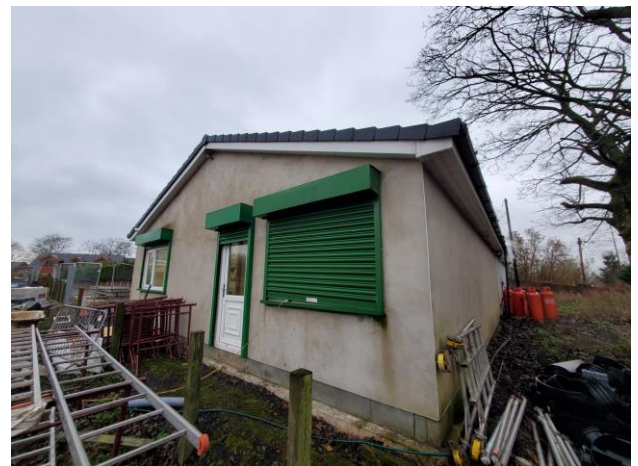
Building on site
