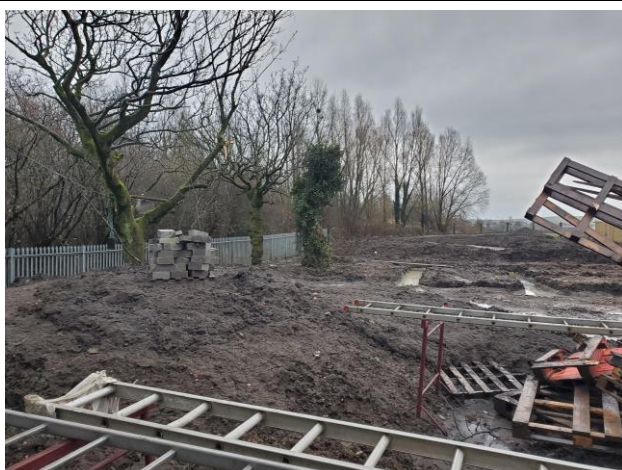
Unvegetated construction area
