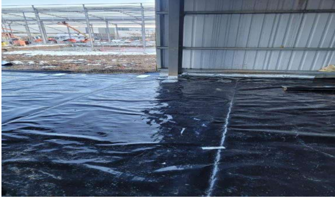
RTEC4 Gas membrane ( Black) RTEC GRSAM (silver) Unit M3 Undercroft
