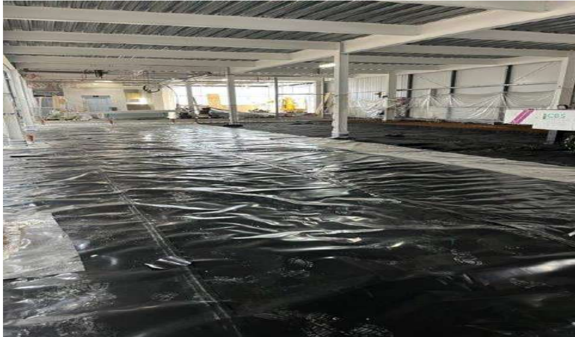
RTEC4 Gas membrane ( Black) RTEC GRSAM (silver) Unit M2 floor areas
