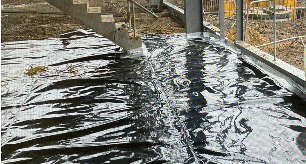
RTEC4 Gas membrane (Black) Unit M1 Undercroft
