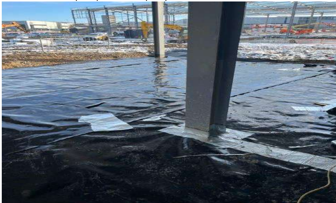
RTEC4 Gas membrane ( Black) RTEC GRSAM (silver) Unit M3 Undercroft
