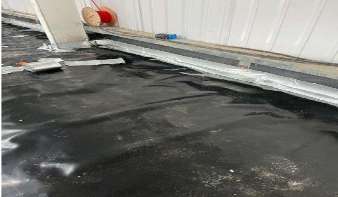
RTEC4 Gas membrane (Black) RTEC GRSAM (silver) to perimeter edge detail Unit M2
