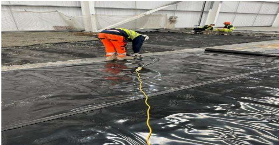
RTEC4 Gas membrane ( Black) RTEC GRSAM (silver) Unit M2 floor areas
