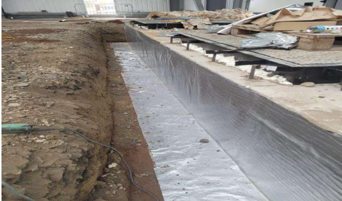
RTEC GRSAM to concrete Docking bays
