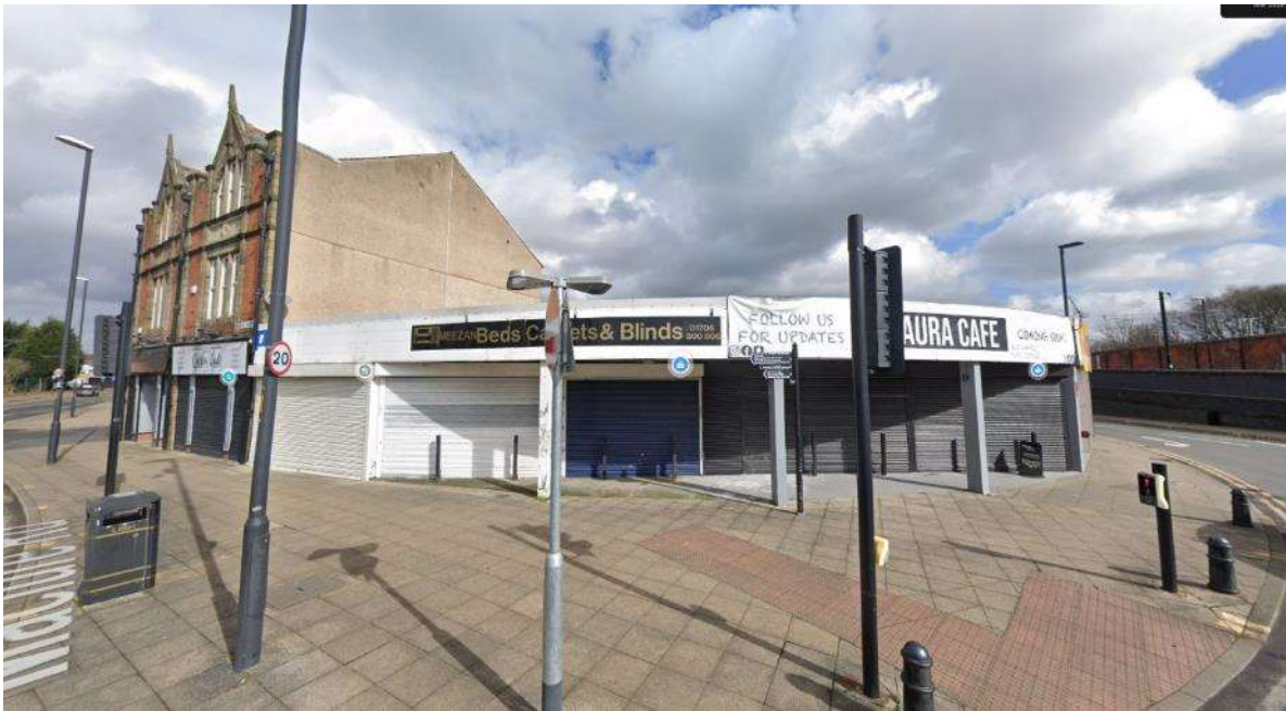
Figure 2 – View on Existing Buildings (Looking North)
