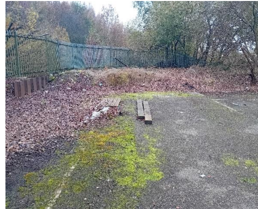
Photo 4: Raised area containing balsam and knotweed at end of hard standing area
