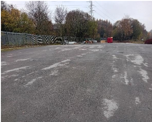
Photo 1: General view of hard standing area
