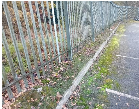
Photo 2: Strip adjacent kerb at base of palisade fence beyond hard standing area
