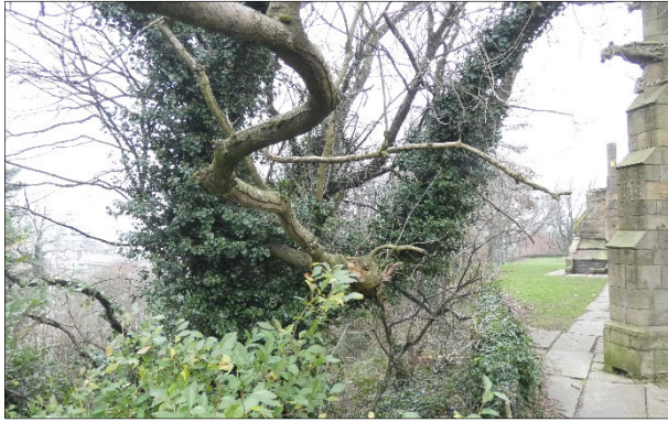
Plate 17. A6T1 South-west facing branch at 5m with lifting bark and an upward facing knot hole. Requires inspection prior to felling .
