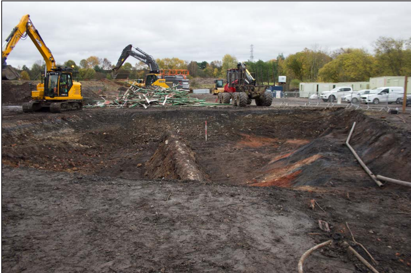
Plate 03: Area 2 post excavation, from the northwest. Scale 2.0m.
