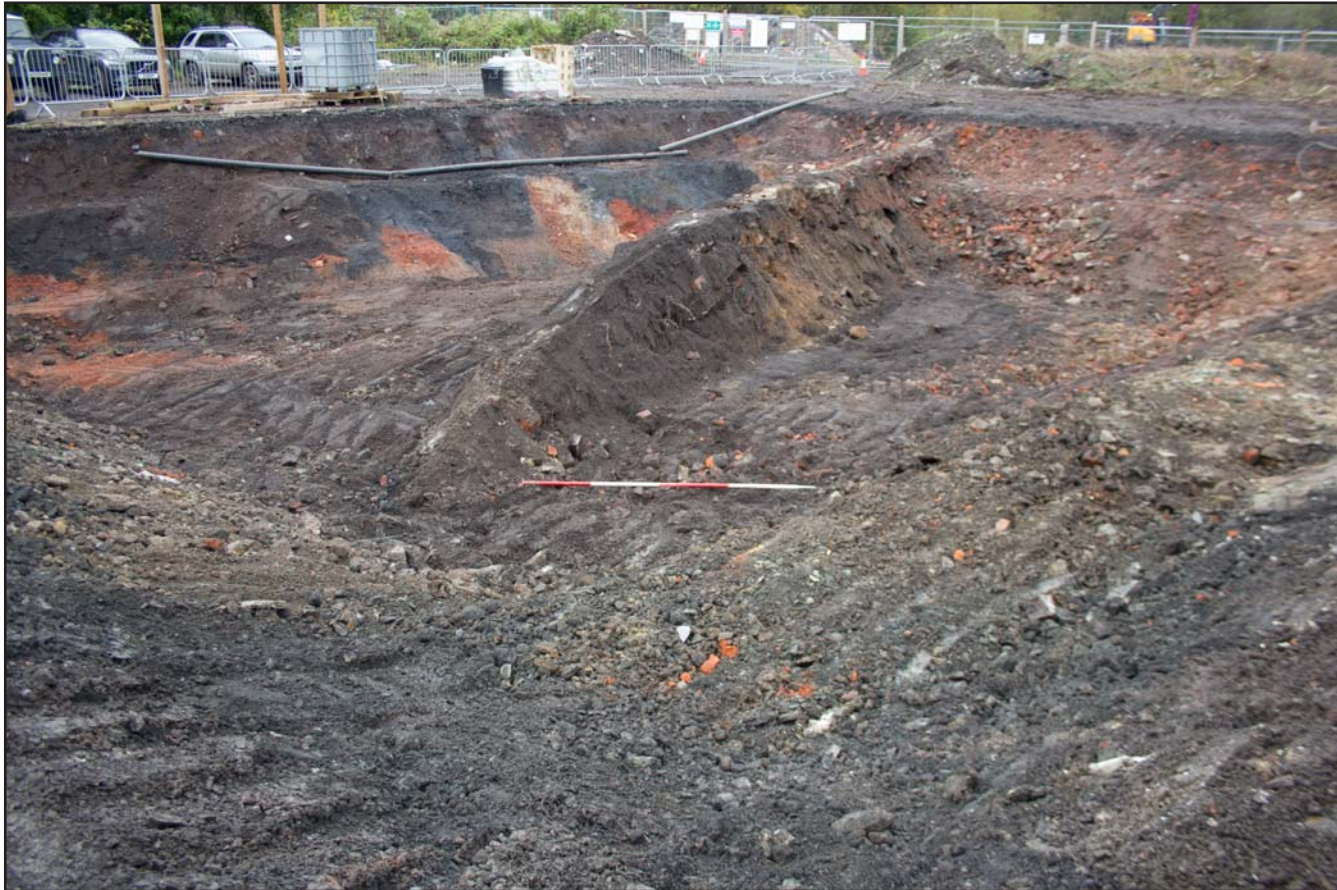
Plate 05: Area 2 post excavation, from the east. Scale 2.0m.
