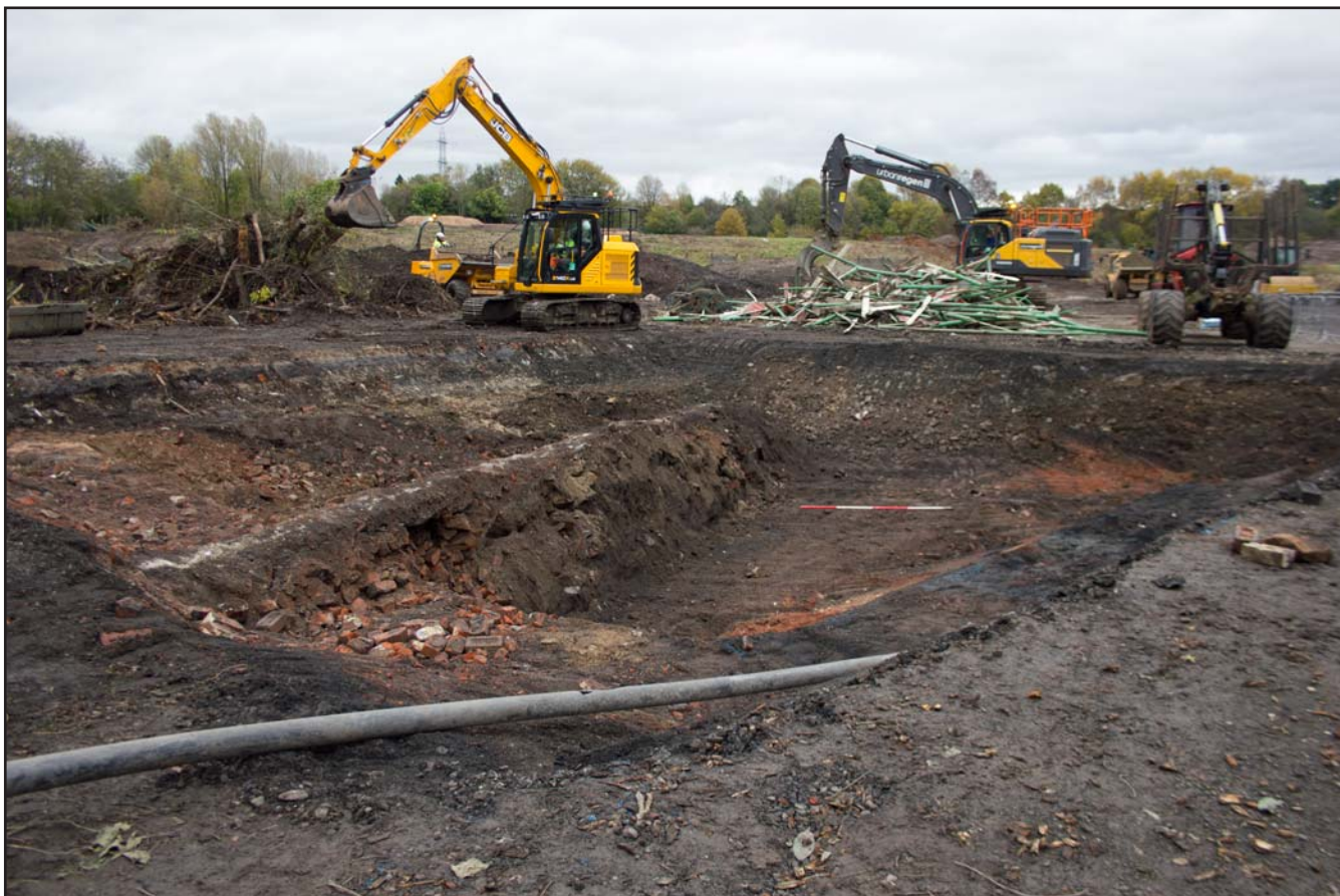
Plate 02: Area 2 post excavation, from the west. Scale 2.0m.
