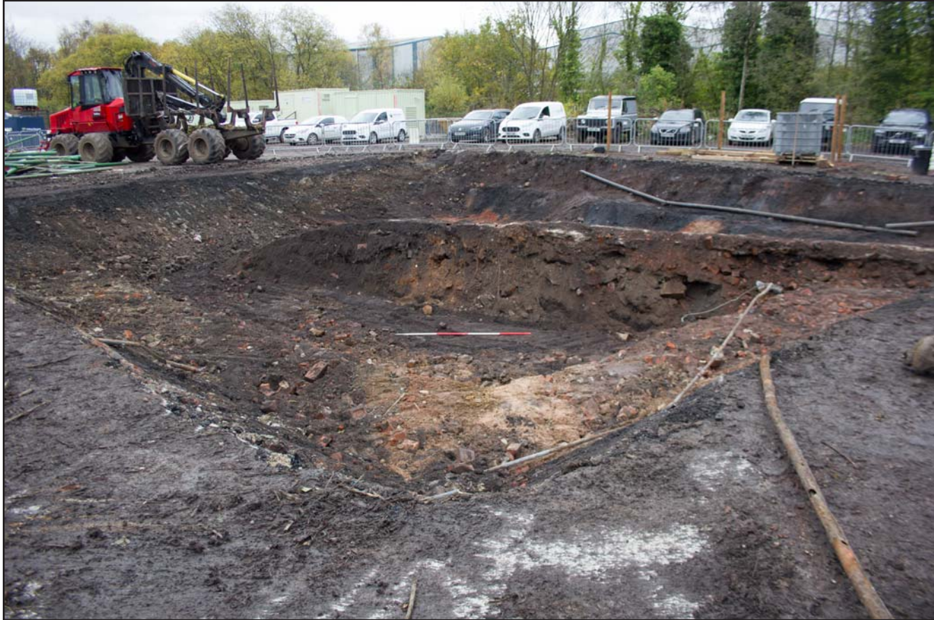
Plate 04: Area 2 post excavation, from the north. Scale 2.0m.
