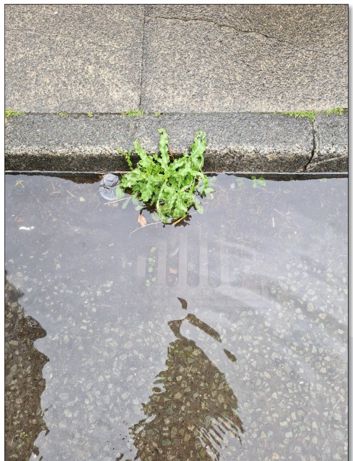
Road Gully Condition Example
