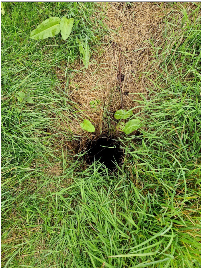
MH3 Location View
