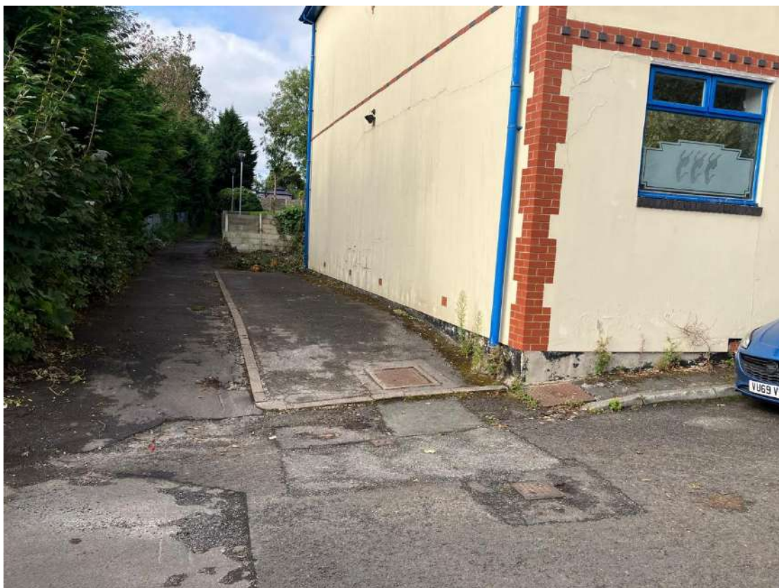
Photograph 2 – Hardstanding to the south-east of the building.
