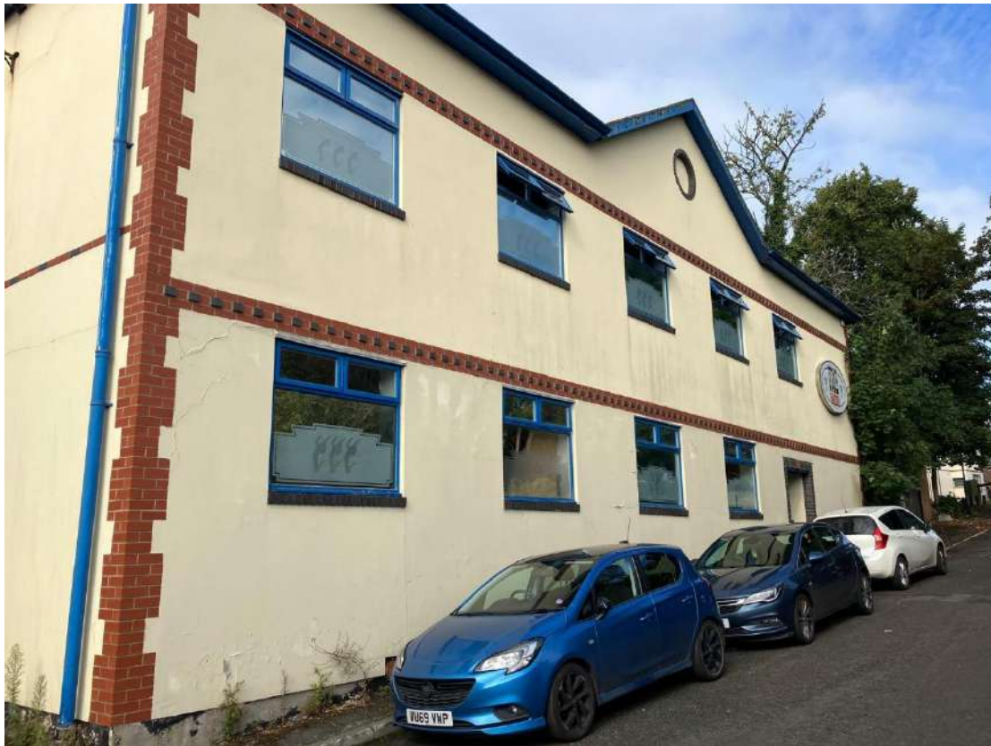
Photograph 1 – Eastern aspect of the building on site.
