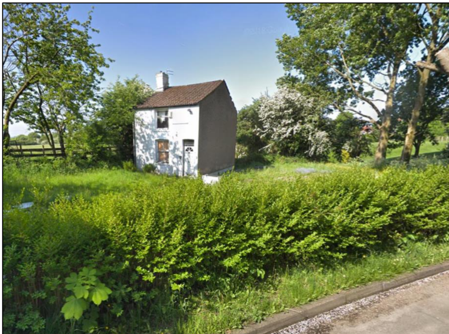
Figure 5: Google Streetview image from May 2018.
