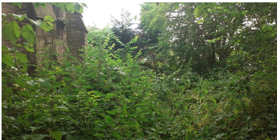
Figure 7 Dense ground vegetation obscuring the church perimeter path
