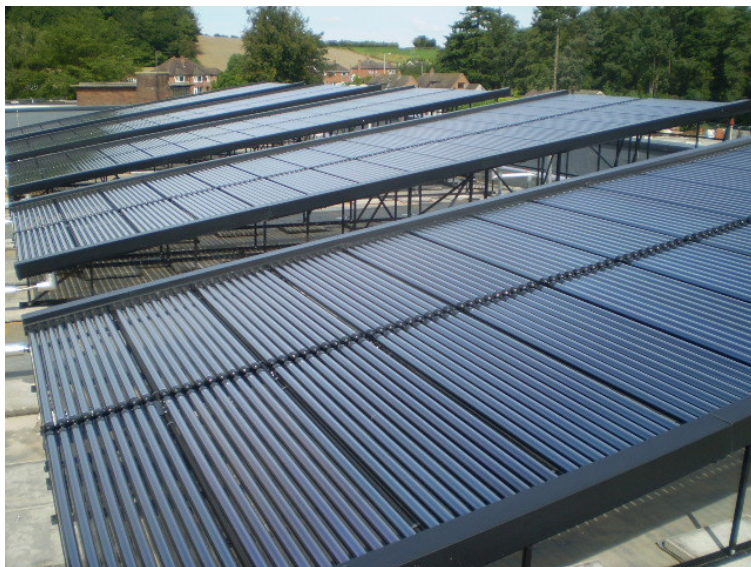
Figure 7. Solar Thermal Evacuated Tube Systems
