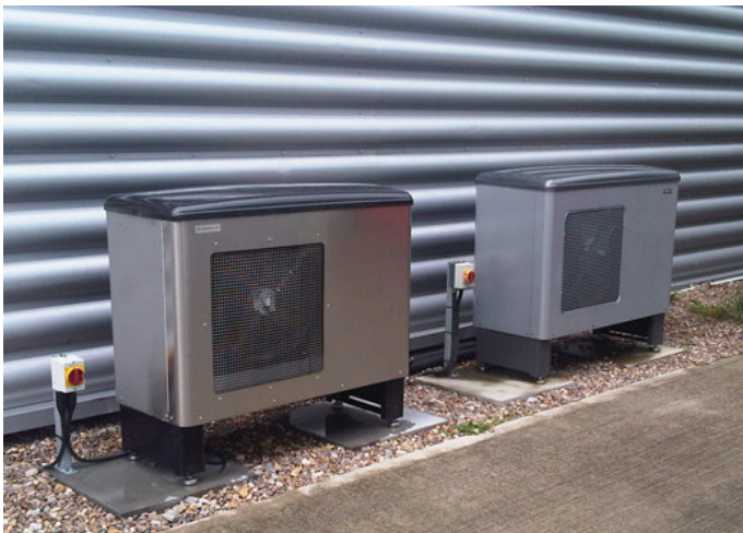
Figure 9. Air Source Heat Pumps
