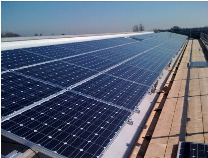
Figure 6. Solar PV Installation
