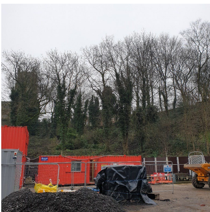
Photograph 5: Area to be cleared with three moderate prf trees, 09:28am. Team were snedding and cross cutting material
