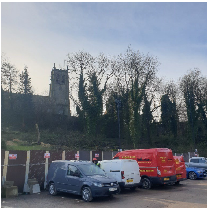
Photograph 1: Working area at end of 01/03/2022
