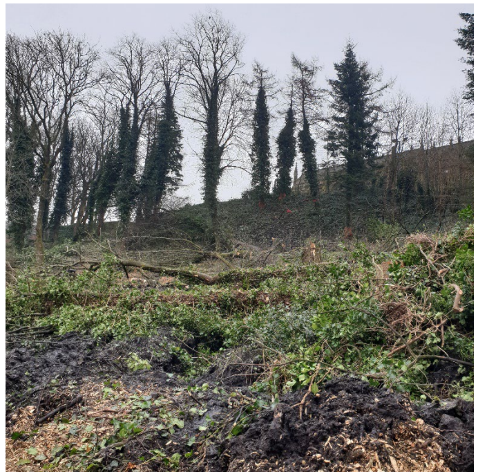
Photograph 2: Two marked up moderate PRF trees (Group) felled on 02/03/2022 prior to ecologist being on site.
