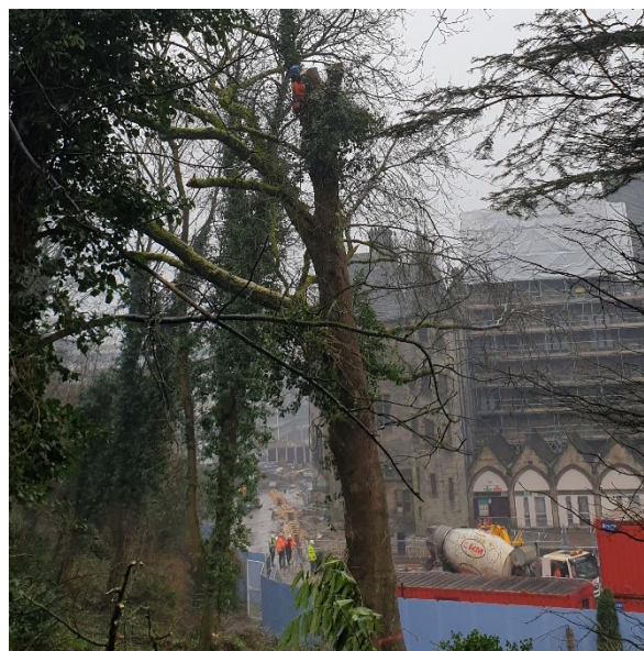
Photograph 4: Ben Stobert and Alex removing Ivy, inspecting features and delimbing standard tree as per requested process, 12:30.
