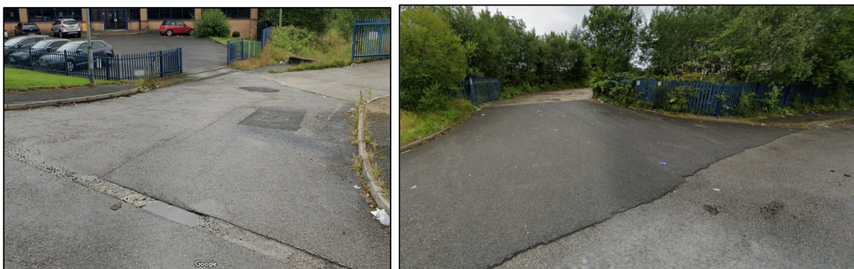
Figure 2.3 – Western Access (Left) and Eastern Access (Right)
