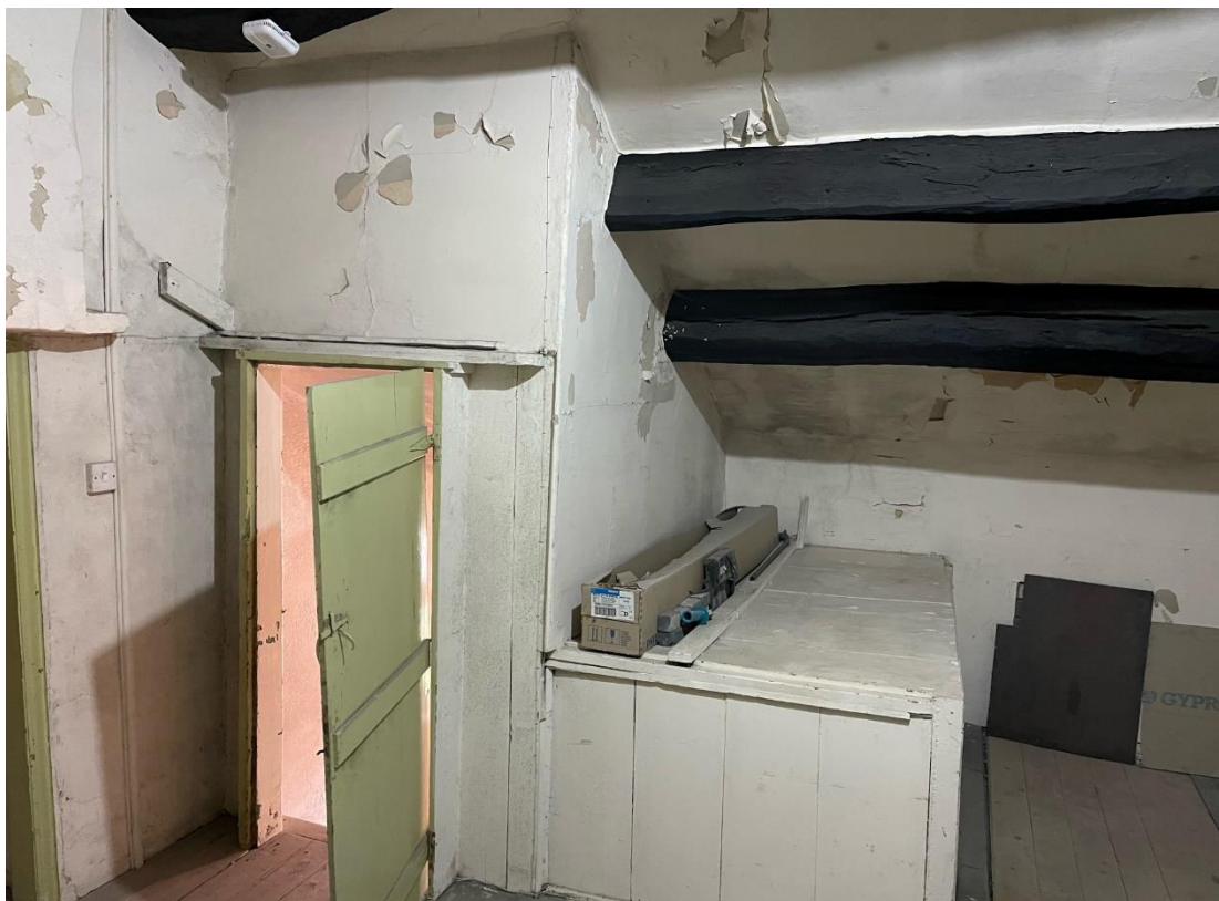
Fig.40: The modern plasterboard bulkhead and door in the attic to be removed.
