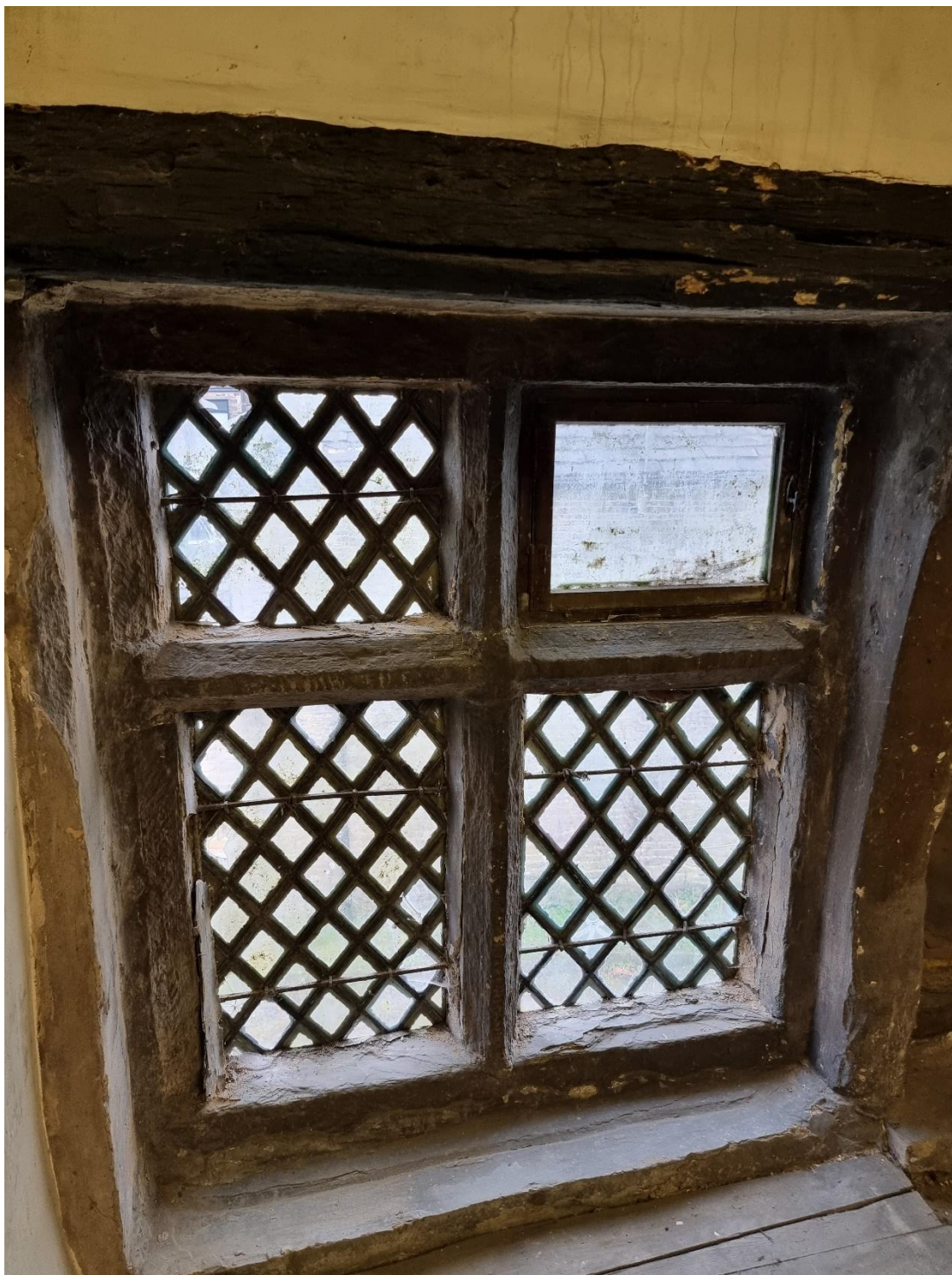
Fig.17: The northeast elevation attic window appears to be contextual with the building, though the top right pane has been replaced with a modern casement..
