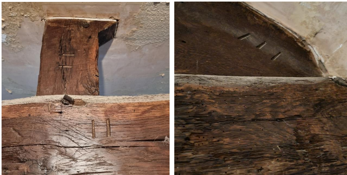
Fig.26: Carpenters marks chiselled rather than scribe into the timber, gives a construction date of post 1700.
