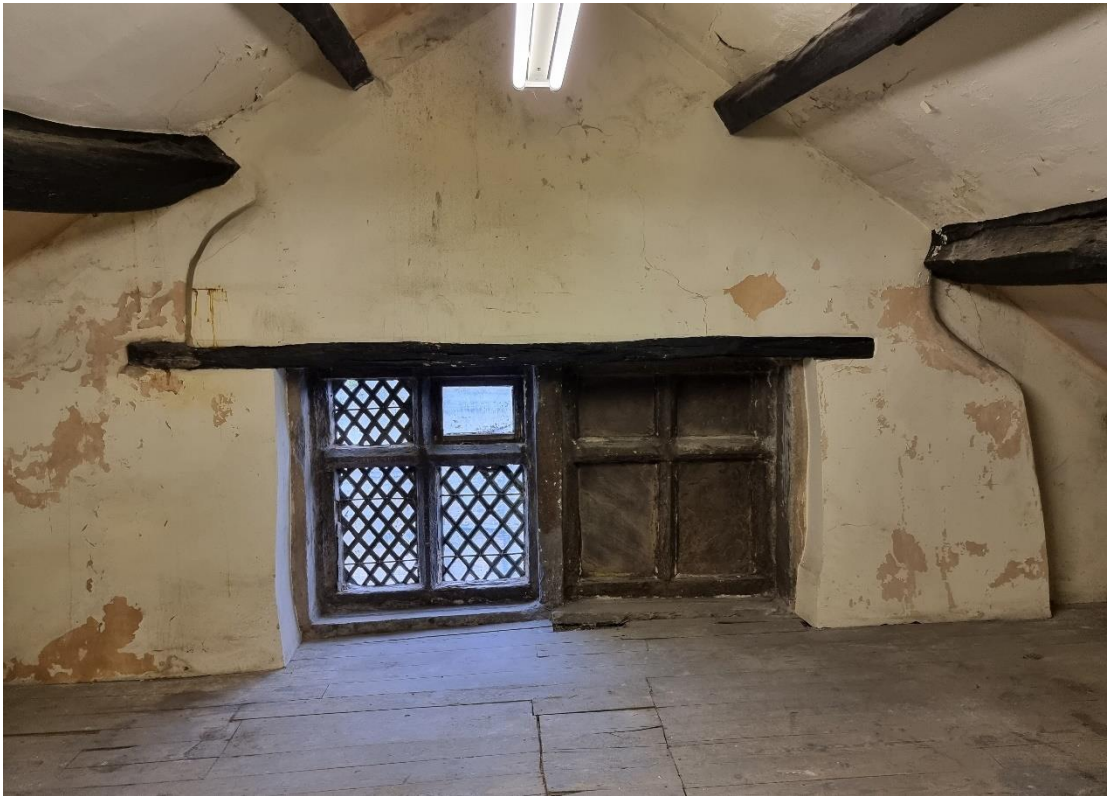
Fig.18: An identical window to the right was blocked in with stone, probably also in the 18 th century in response to the window tax in force at the time. This corner of the building is the oldest part of the house, and the historic beams can also be seen in this image.
