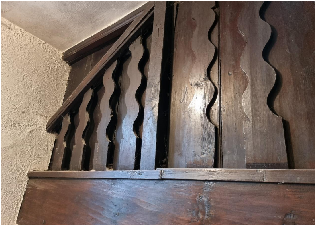
Fig.19: 'Splat' balusters such as these date to the early 18 th century, suggesting they are an original feature of the house.
