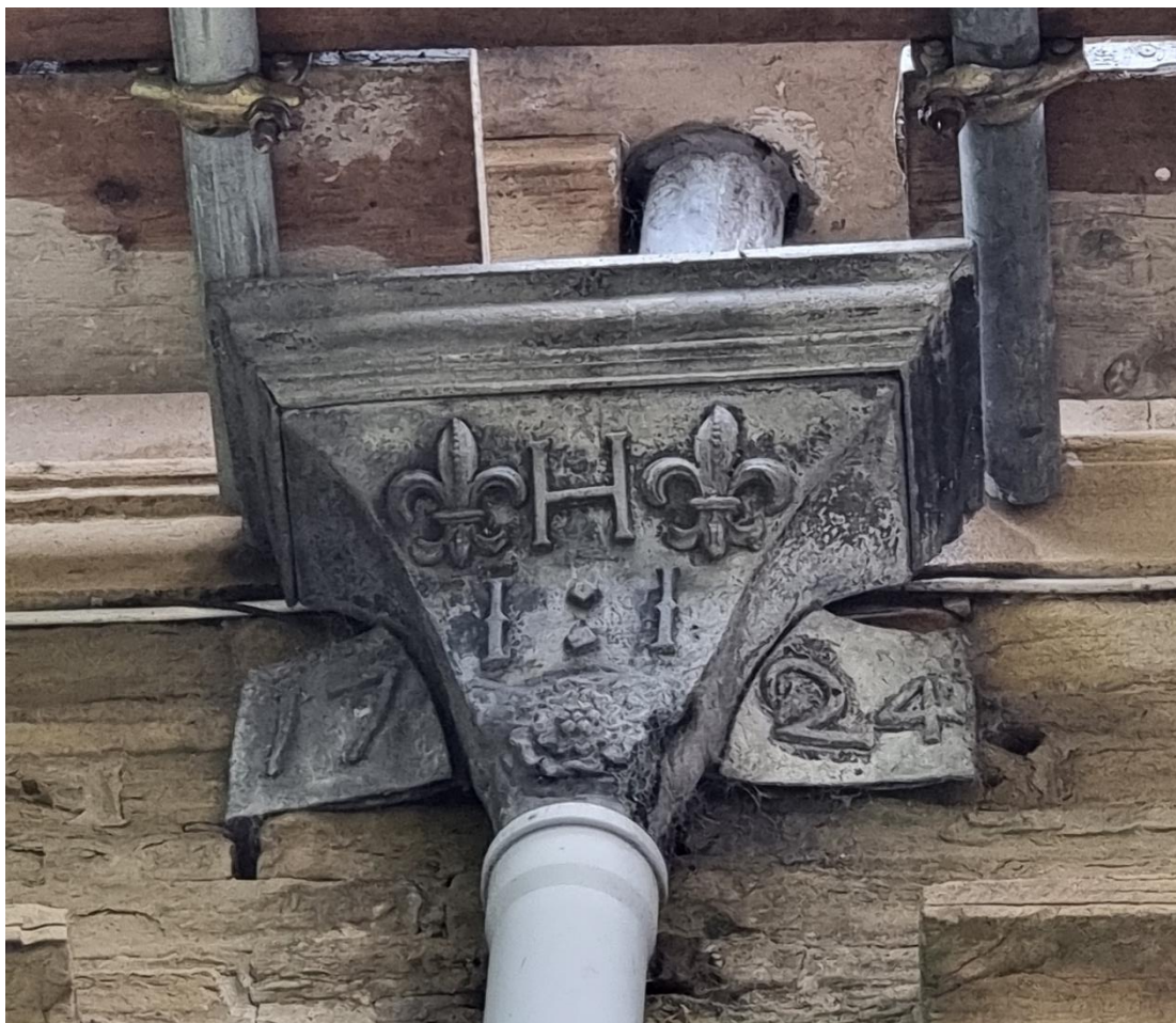
Fig.16: The rainwater hopper stamped with the date 1724.
