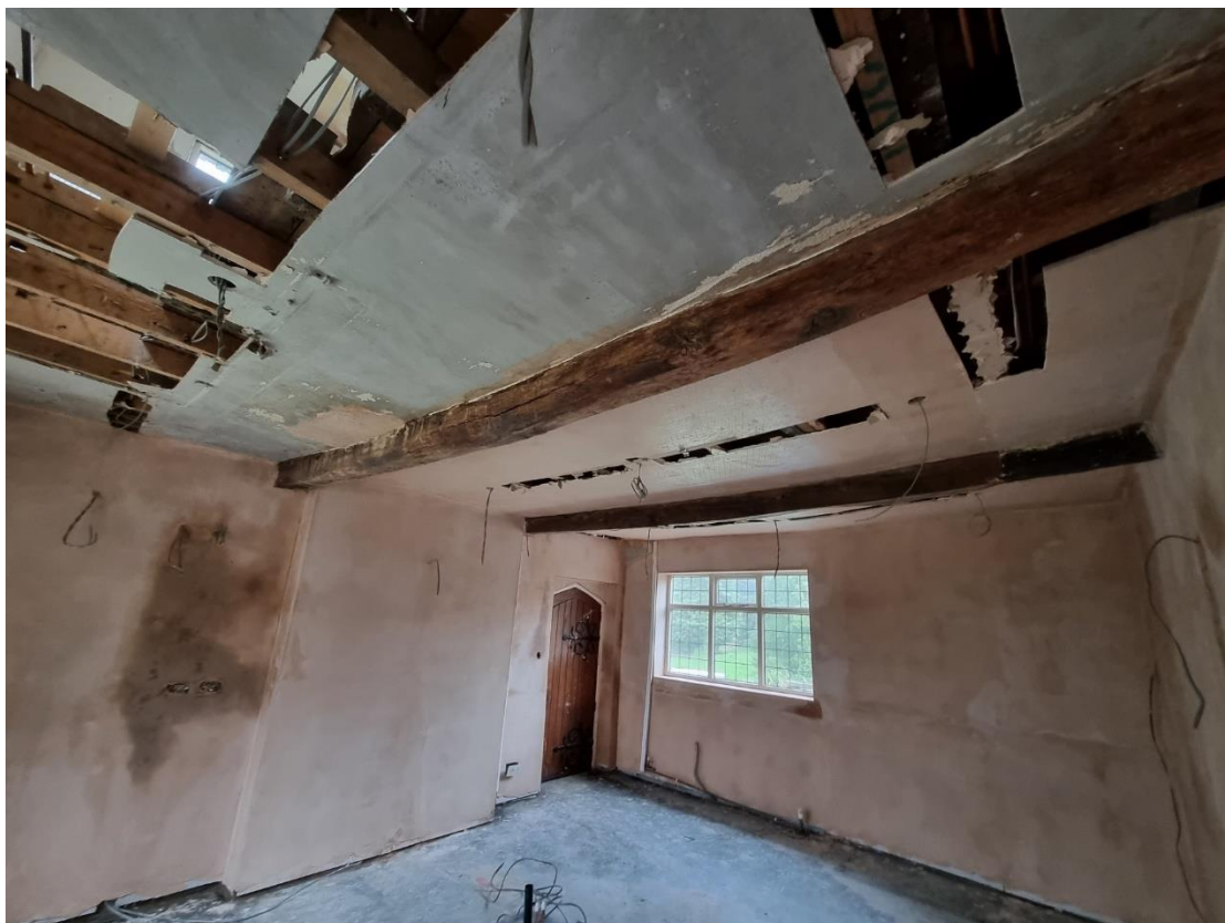
Fig.29: Gypsum plasterboard to kitchen to be removed and replaced with lime mortar
