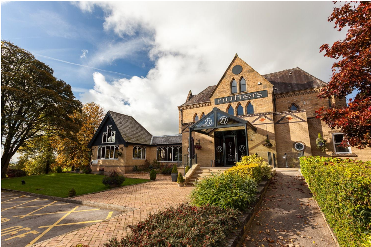
Figure 7. Image of the principal south facing elevation. The modern extensions project forward of the host building.
