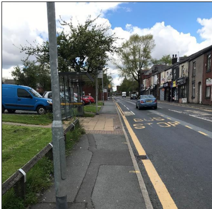
Figure 10. Northbound bus stop along A671 Whitworth Road
