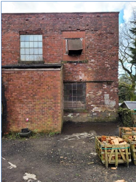
Photo 1. shows the existing condition of the staircase location.
