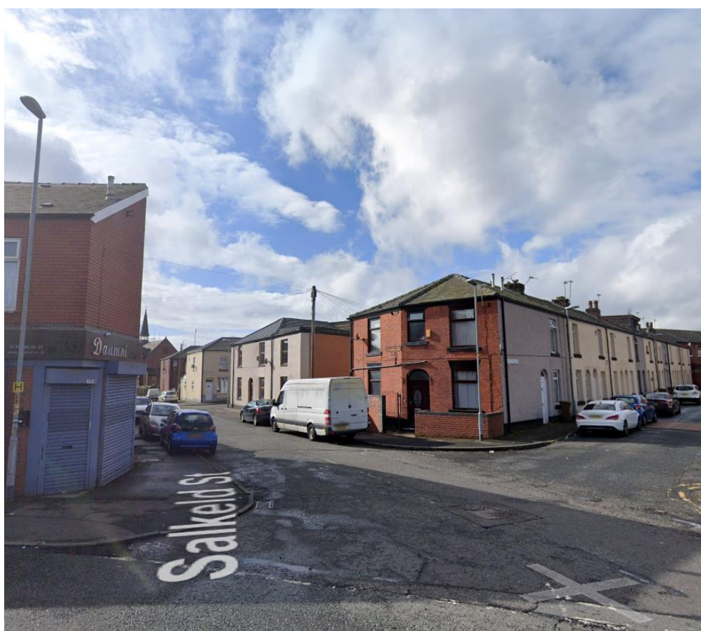
Above: Image shows the gable front elevation of the application property .
