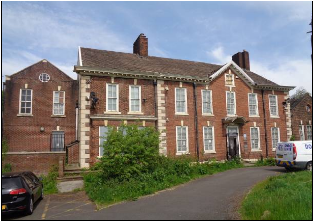
1. The fine early Classical front elevation of the listed building
