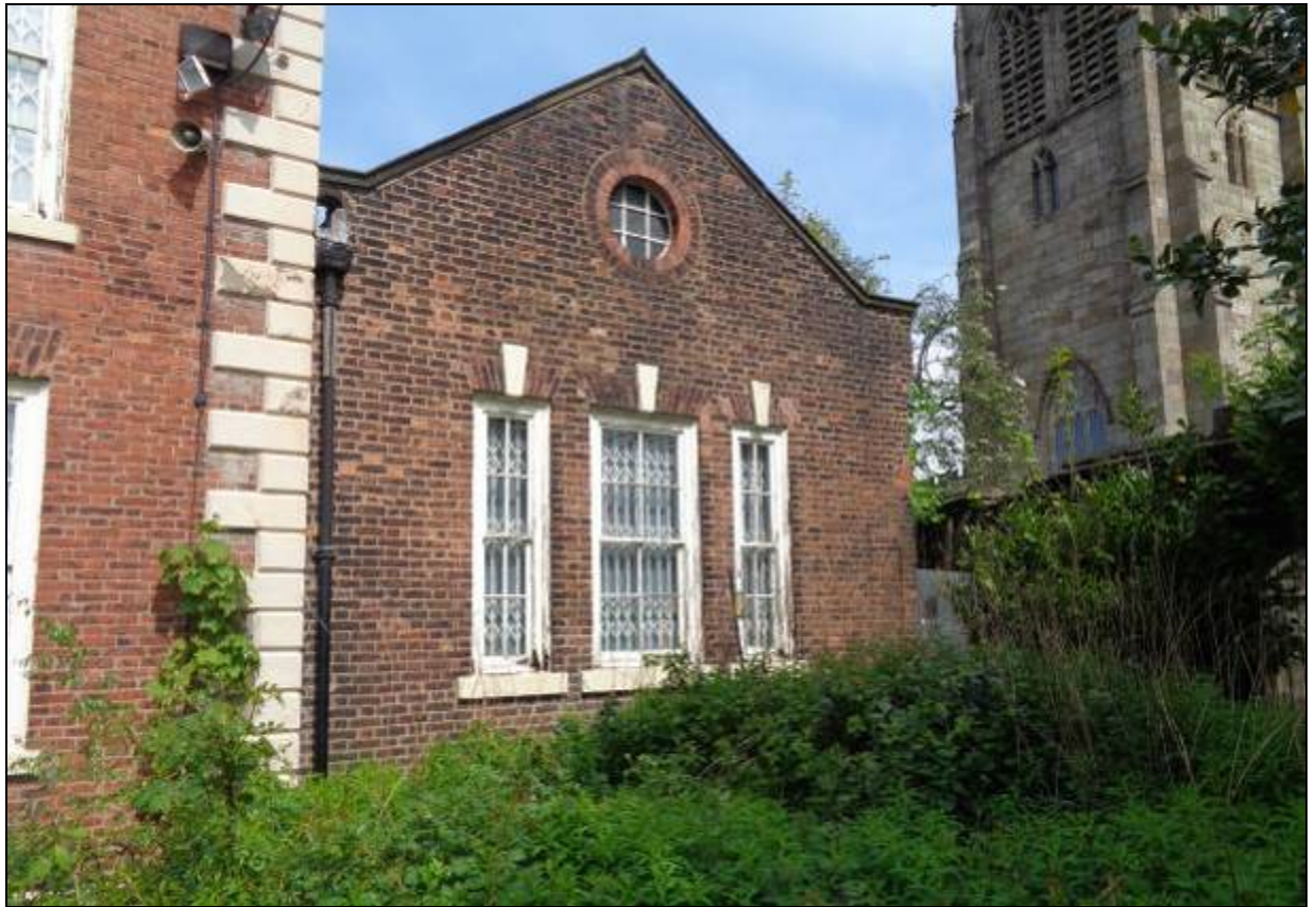
19. Front elevation of the late 19 th century wing
