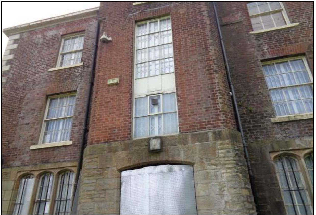
9. Stair tower appears rebuilt probably in the mid-later 19 th century
