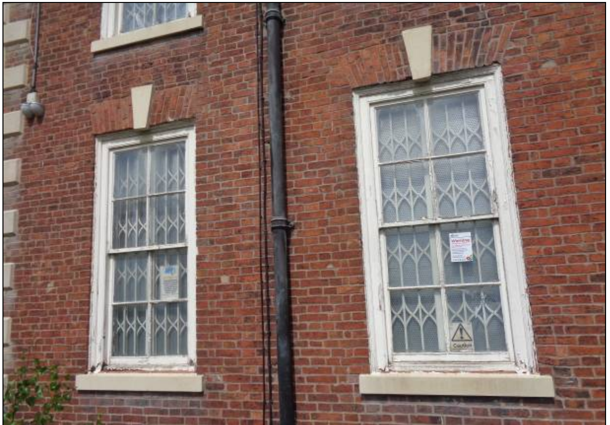
7. Window framing is probably mid-20 th century
