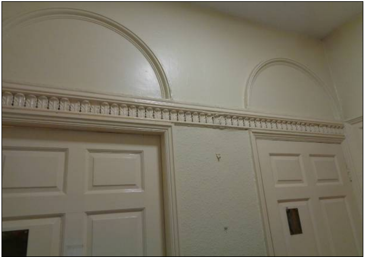
13. Relocated panelled doors and frieze on first floor
