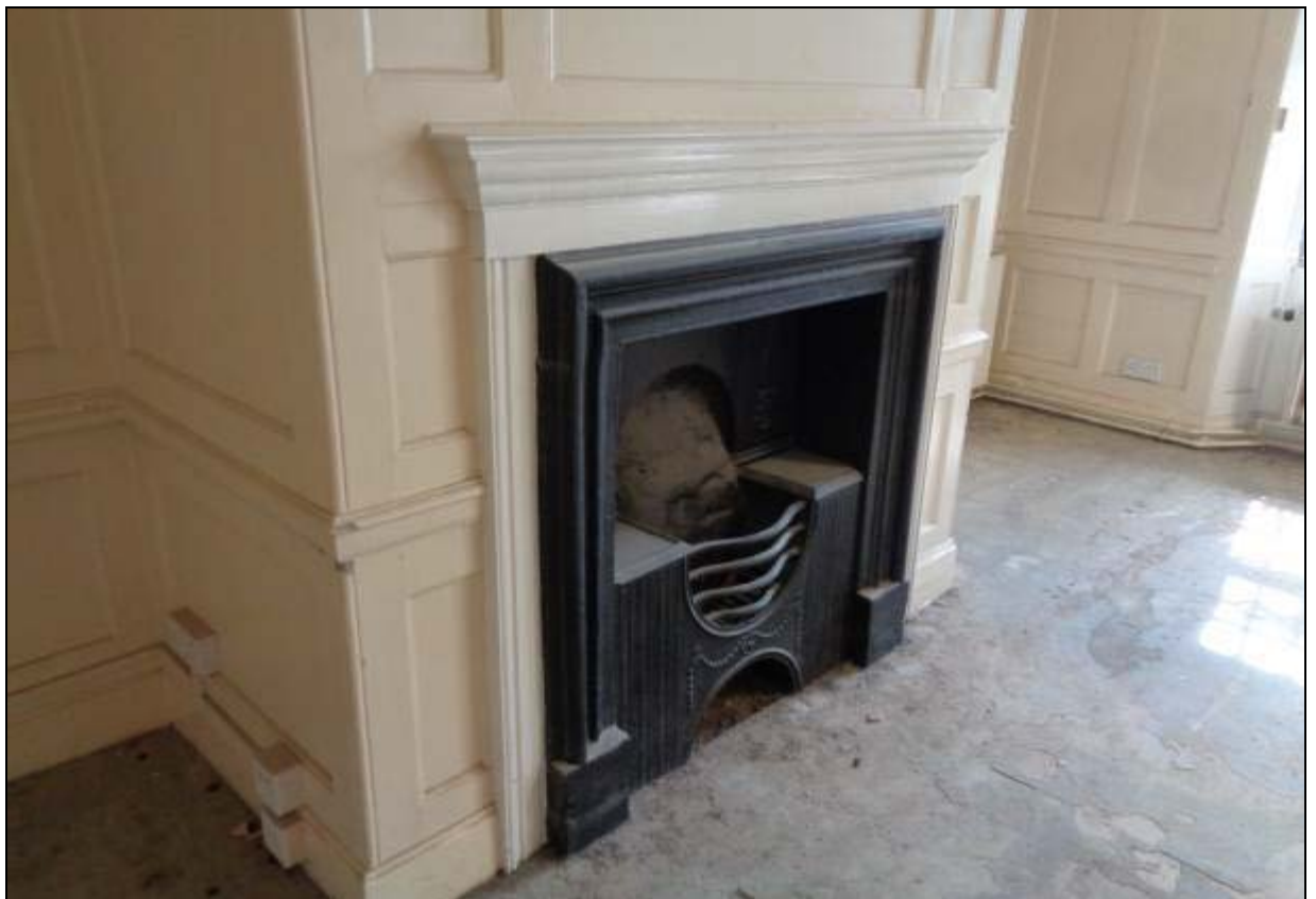
14. Late 18 th /early 19 th century hob grate in first floor right front room
