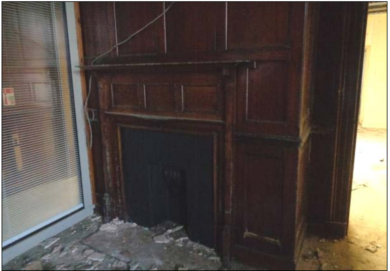
11. Panelling and fireplace in rear right room, early 20 th century
