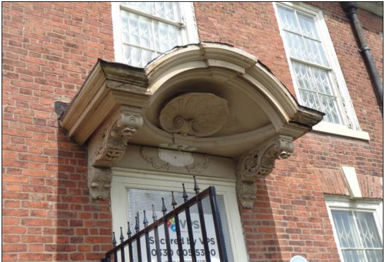
6. The door canopy is however early 20 th century
