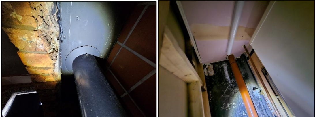
Photographs 23 (left) and 24 (right) showing the interior of the chimney and boiler room, respectively.
