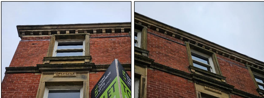
Photographs 4 (left) and 5 (right) showing modillion cornice and window frames.
