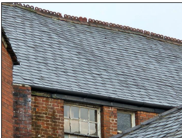
Photograph 6 showing a detail of the rear elevation.
