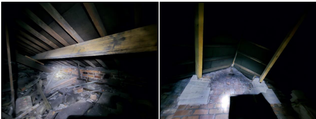
Photographs 9 (left) and 10 (right) showing the interior of the roof space.
