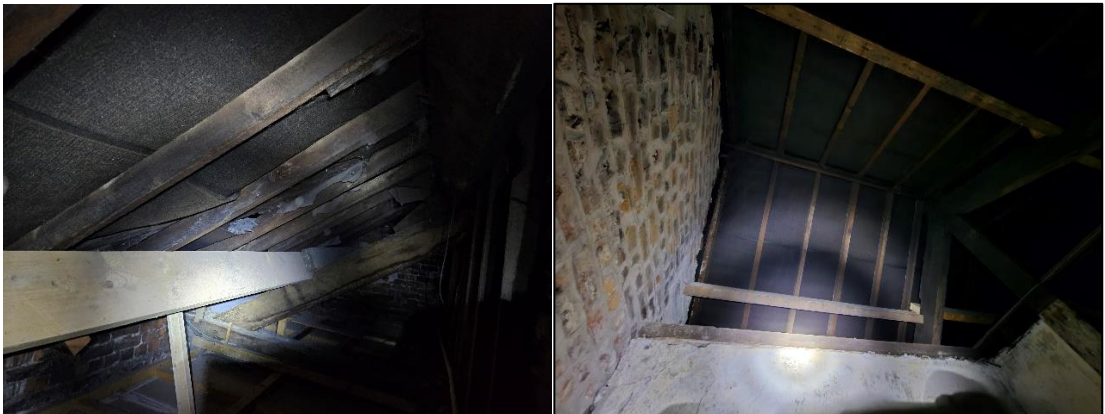
Photographs 13 (left) and 14 (right) showing the interior of the roof space with wooden beams and membrane, and gap at gable end, respectively.
