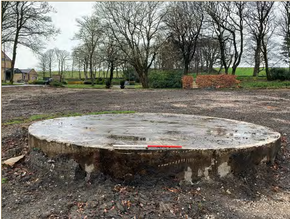
Photograph 15: View towards concrete circle foundation.
