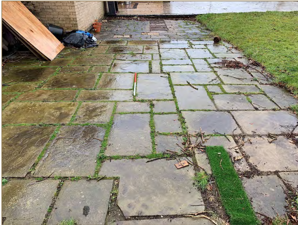
Photograph 9: View of possible original flagged area.
