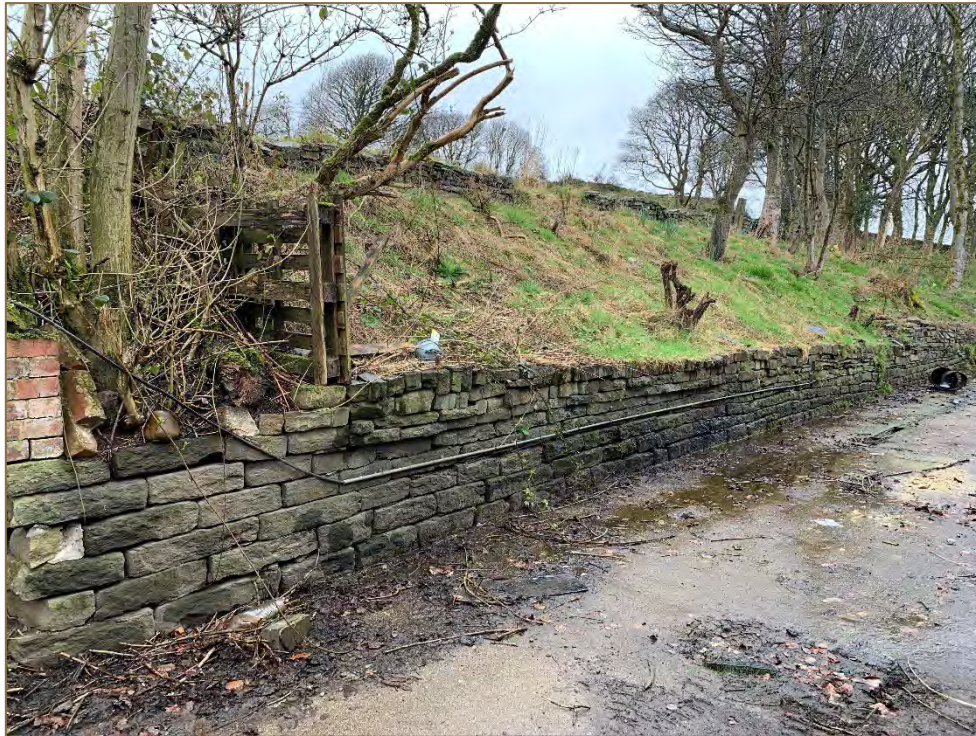
Photograph 7: View northwest over the PDA, dry stone wall embankment.
