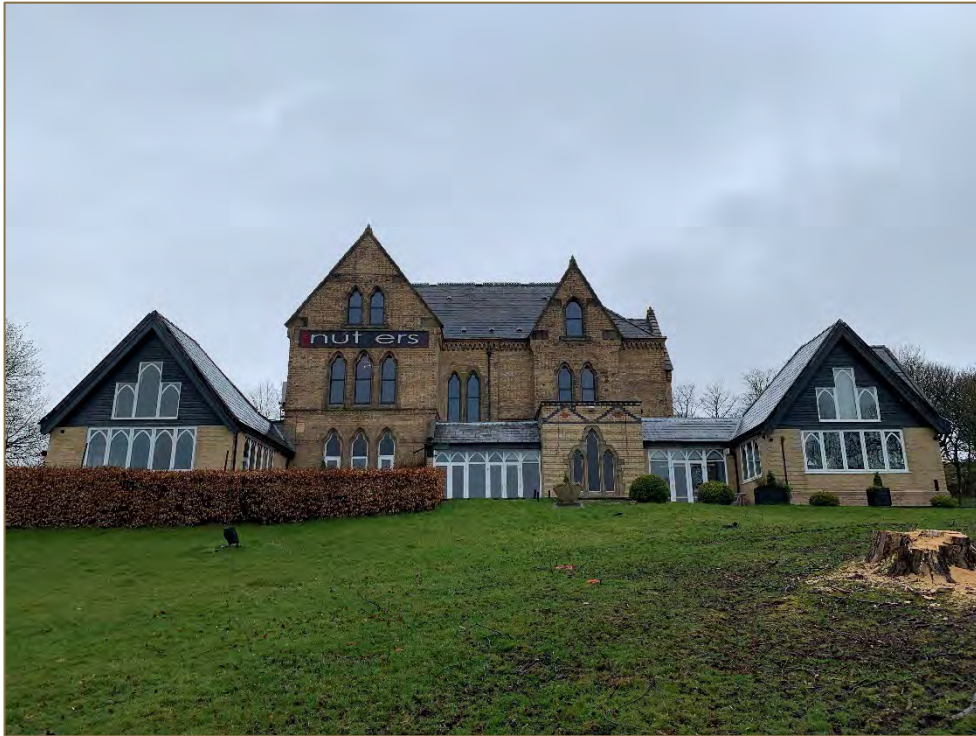
Photograph 1: View north towards the former Nutter's Restaurant Building
