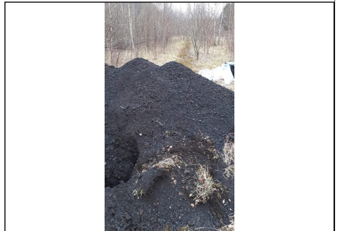
Trial Pit 117 Spoil
