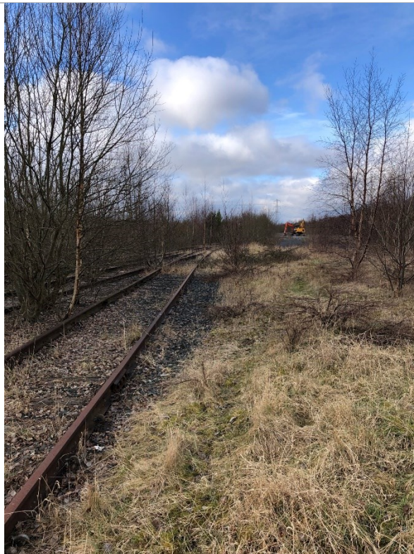
PLATE 2 VIEW OF SITE FACING NORTH THROUGH CENTRE OF SITE
