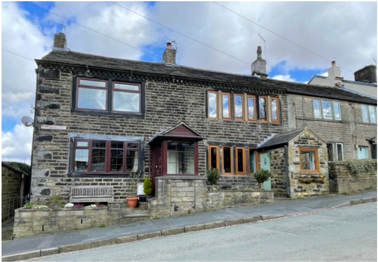
Existing front elevation showing existing porch to No1 and the porch to No 3 that the client wants to replicate to the front elevation of No1
