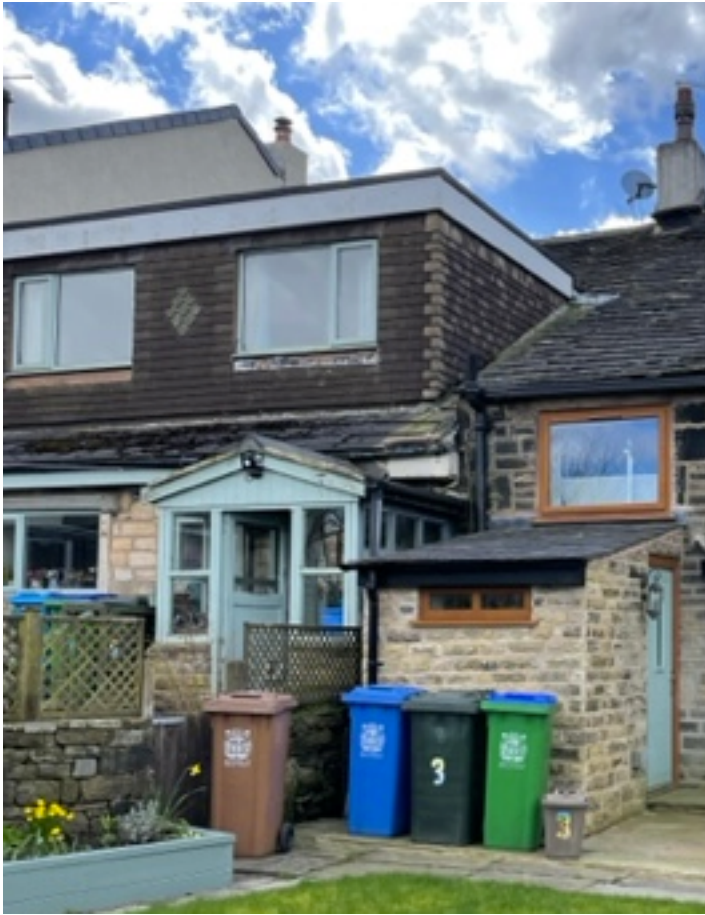
Existing rear elevation image of No 5 showing various extensions and alterations with part of No3 to the right
