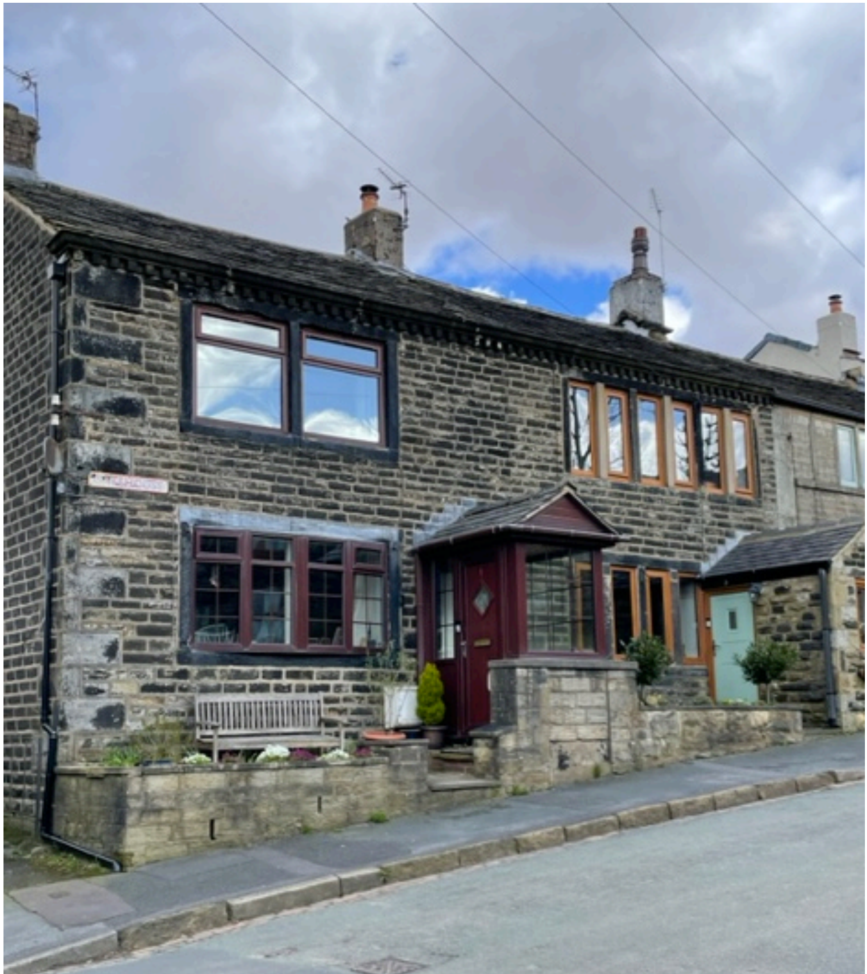
Existing front elevation showing side return wall where client would proposes to form new stepped access from garage to the left of the dwelling
