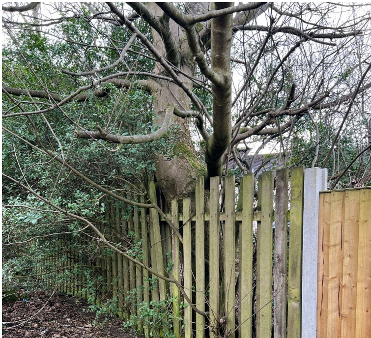
Photo 2: T1 and damage to boundary fence.
