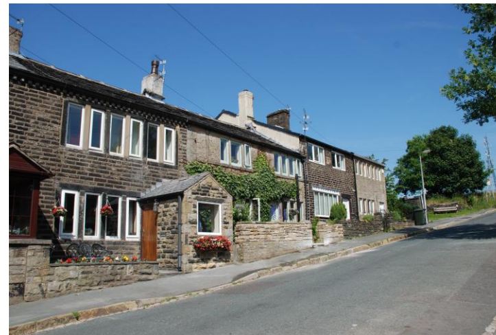
cottages to the east of the site
