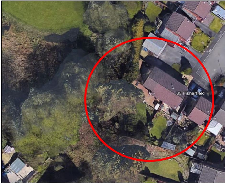
Fig 4. Aerial image of 33 Fisherfield, Rochdale.
