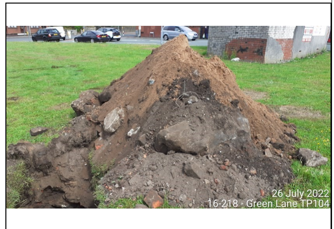
Trial Pit 104 Spoil
