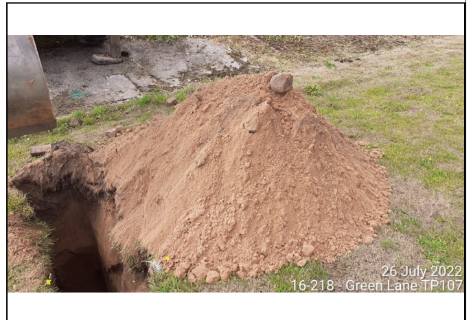
Trial Pit 107 Spoil
