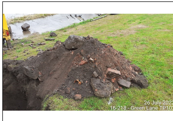
Trial Pit 103 Spoil
