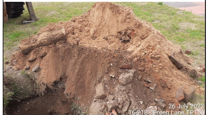
Trial Pit 106 Spoil
