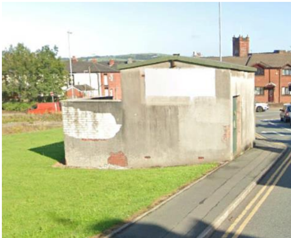
PLATE 4 SUBSTATION PRESENT ALONG THE EASTERN BOUNDARY OF THE SITE
