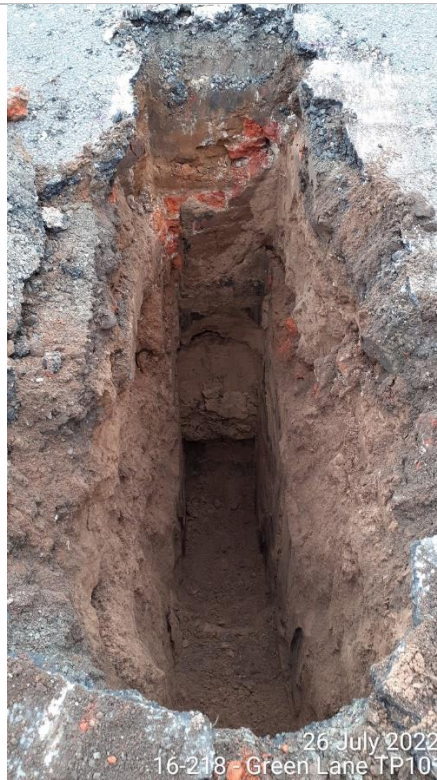
PLATE 2 SAND PRESENT UNDER HARDSTANDING - WESTERN SECTOR OF SITE
