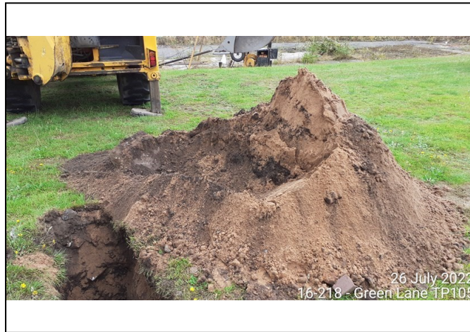
Trial Pit 105 Spoil
