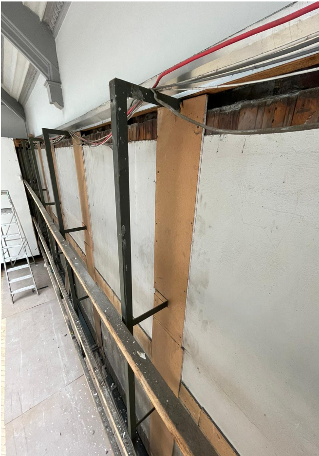
Image 02/04 - Closer look at existing Steel/Timber substructure, installed to hold the contemporary exhibition boards.
