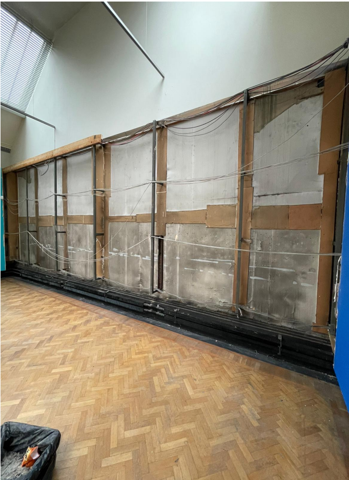
Image 04/04 - Timber battens elements removed leaving steel structure fixed to original brickwork walls.
