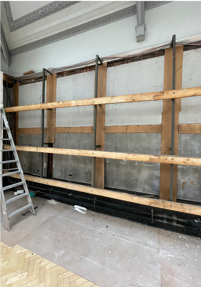
Image 01/04 - Section of Exhibition boarding removed to reveal location of typical vent (gallery 04). However, a further board has been installed over the original T&G to block openings.
