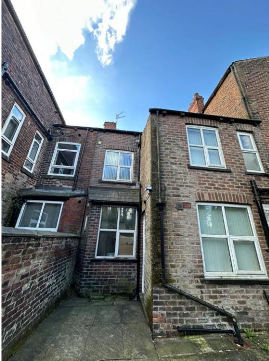
Rear elevation of No 20 Mellalieu Street
