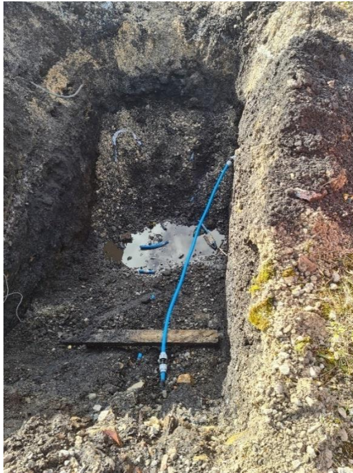
PLATE 3 REPIARED WATER PIPE (TP402)
