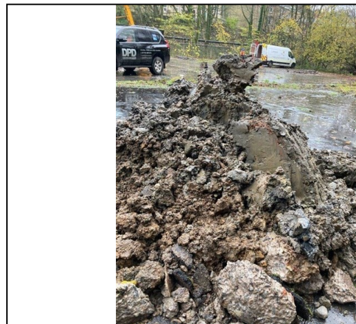
Trial Pit 125 Spoil
