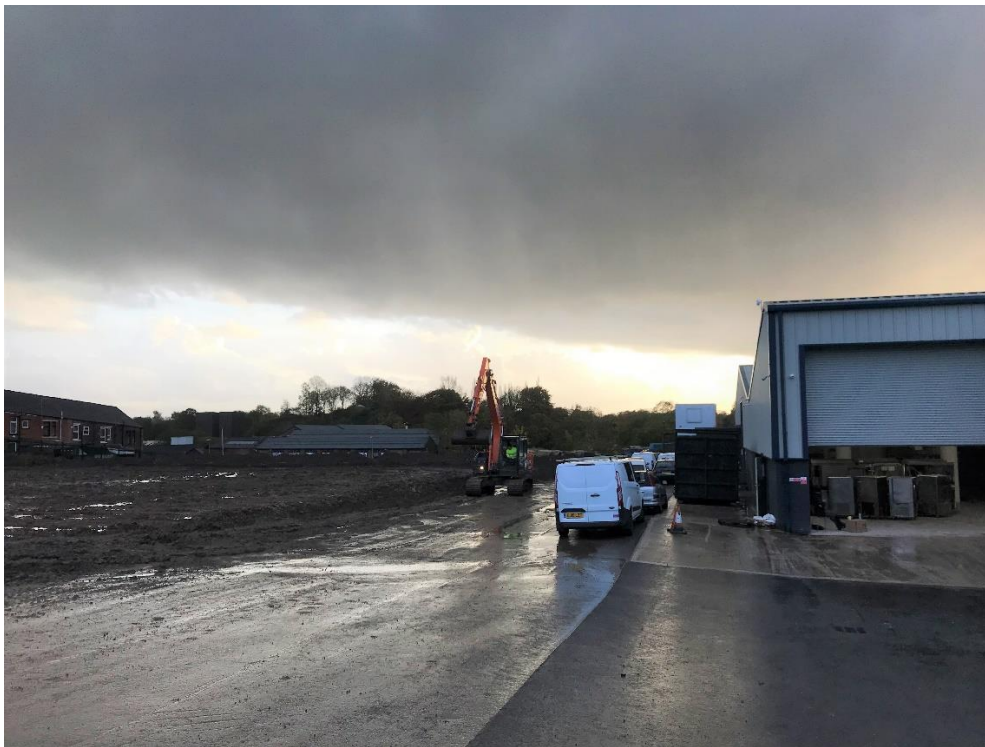
Figure 2.4: Photo looking south across the cleared site, the existing commercial unit is within the right of the view.
