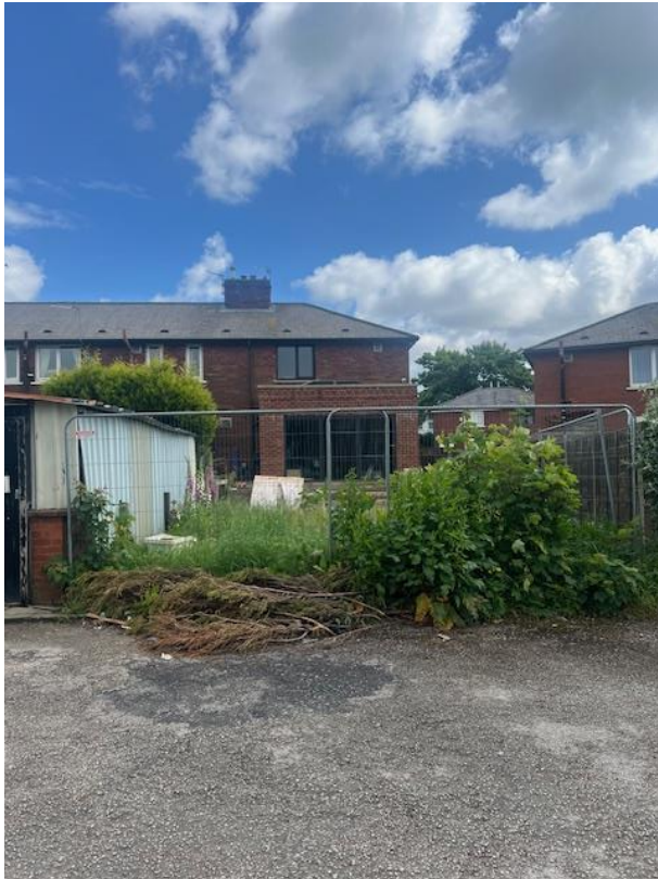
Rear elevation of application site
