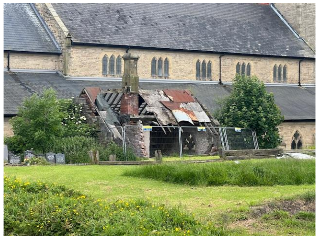
North eastern elevation of former meeting room
