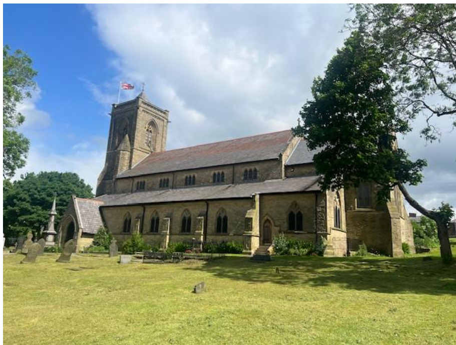
St James's the Apostle Parish Church (south western elevation)
