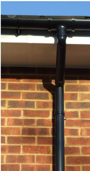
Black Colour Round Plastic Pipes and Half Round Gutters.
