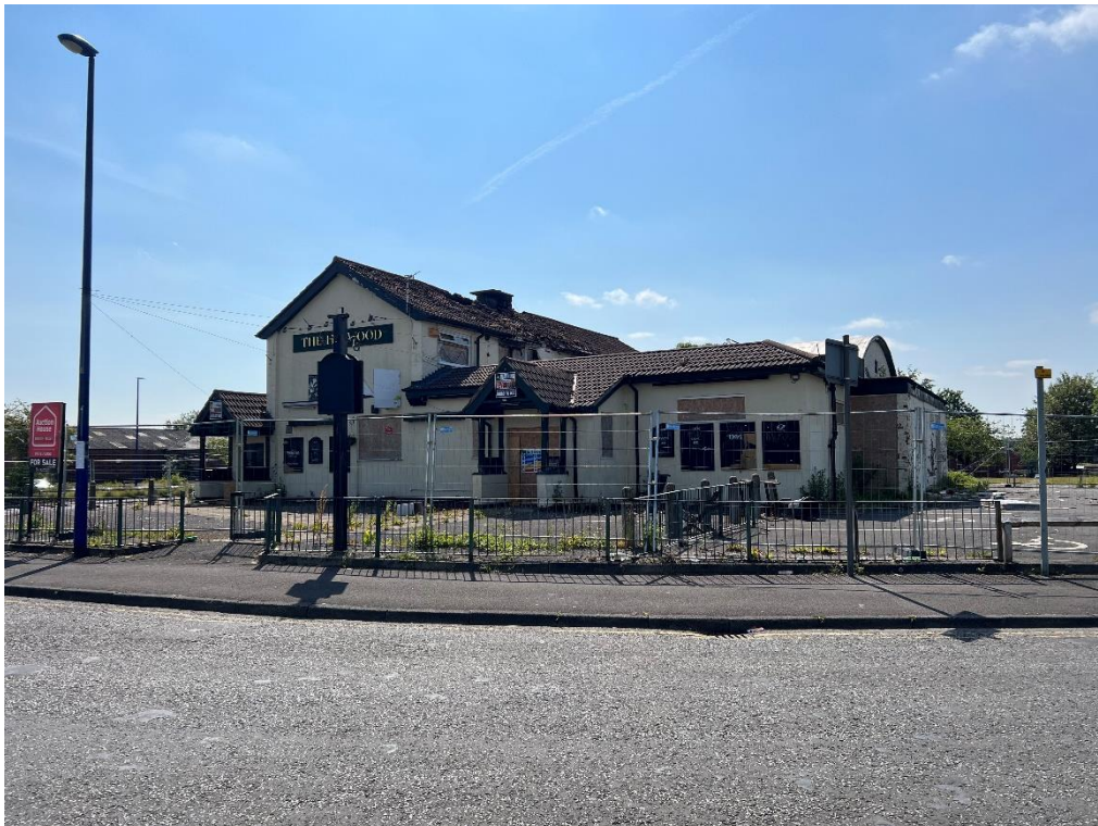
The Heywood public house before demolition (June 2023)
