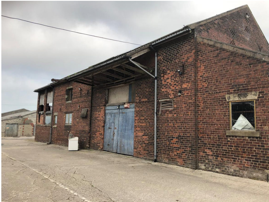
Figure 4.10: Barn forming part of the U-shaped farmyard
