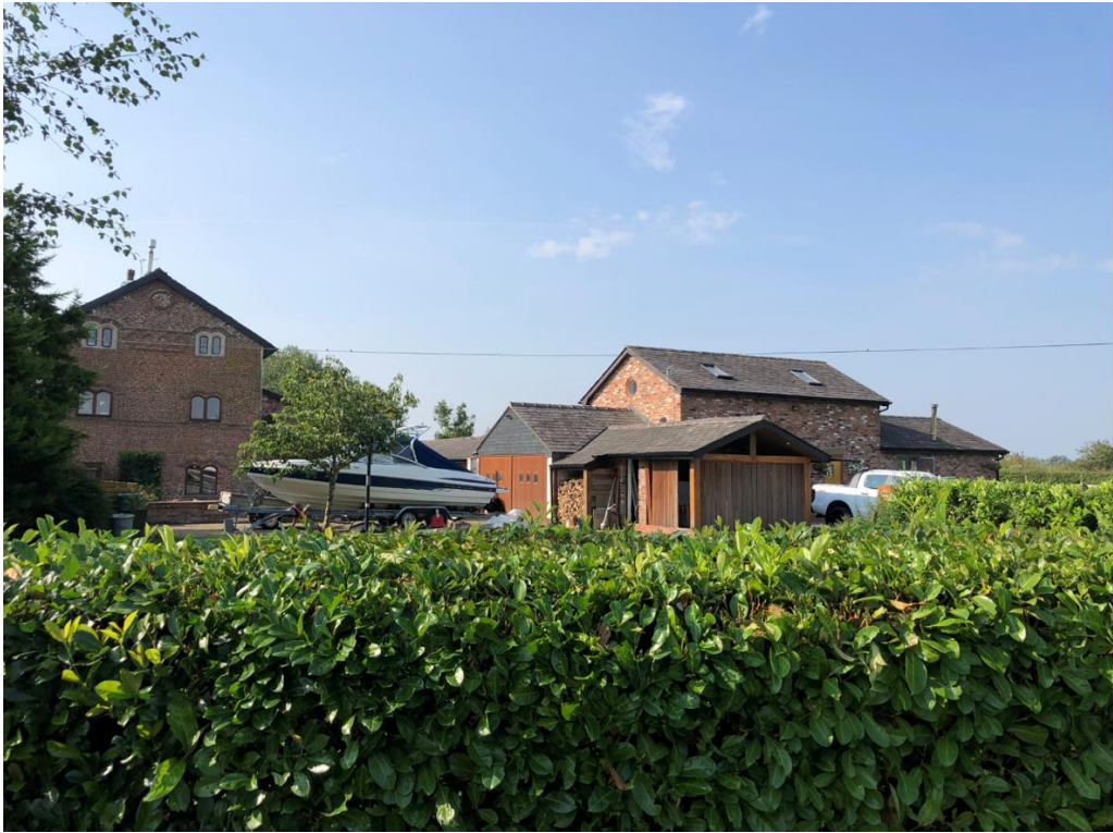
Figure 4.6: South elevation of Brick Farmhouse (left) with later additions and outbuildings (right)
