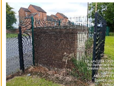
Built structure in the west of the site
