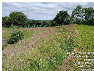
Embankment in the west of the site
