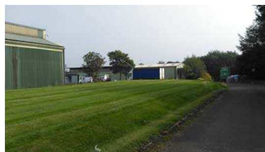
Unit B on left with raised grassed area in foreground and Unit G in background and pallets on far right
