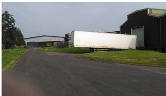
Unit B on right with scaffolding poles stored to the north and Unit A (off site) in background
