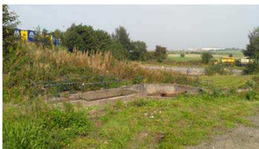
Redundant sewage settlement tanks (off site), looking northeast away from the site
