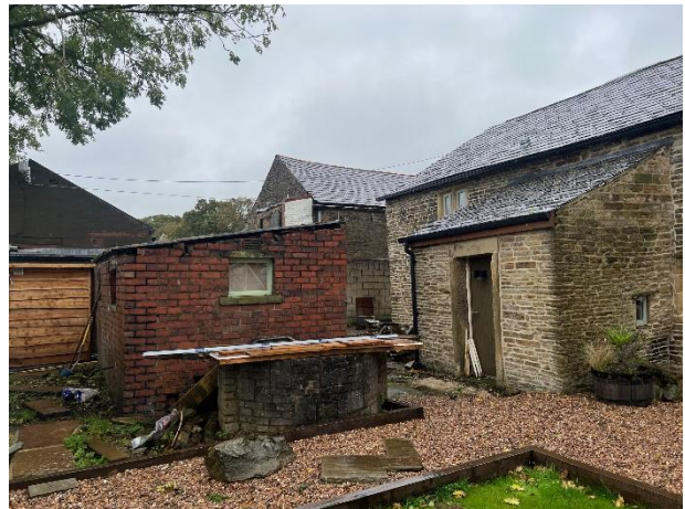
Lean-to porch, well and brick outbuilding
