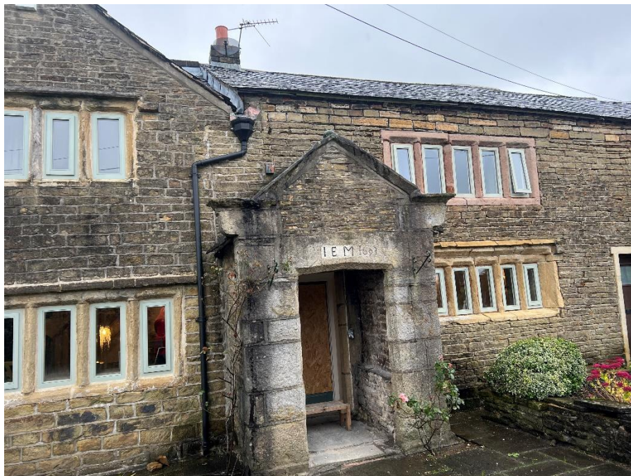
Date and initials to porch lintel
