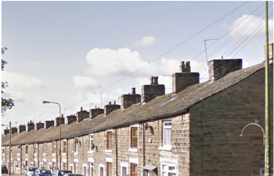
Long continuous sloping terraces with consistent chimneys (Hadfield)
