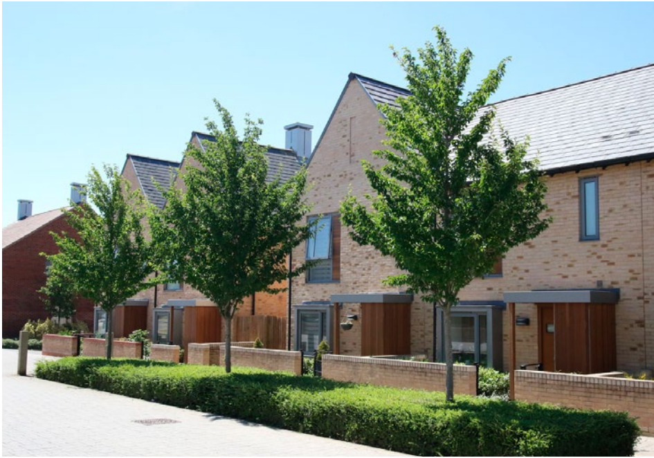
Local gritstone and timber responding to existing materiality
