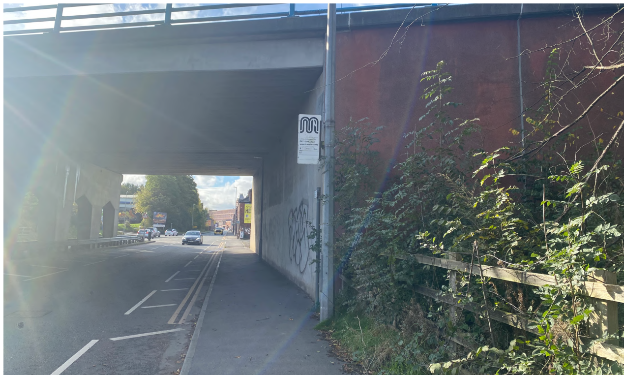
Photograph 2.2 : A664 (Queensway) - Bus Stop
