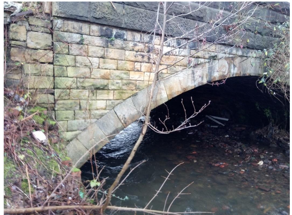
Figure 14 Bridge as viewed from the Site.
