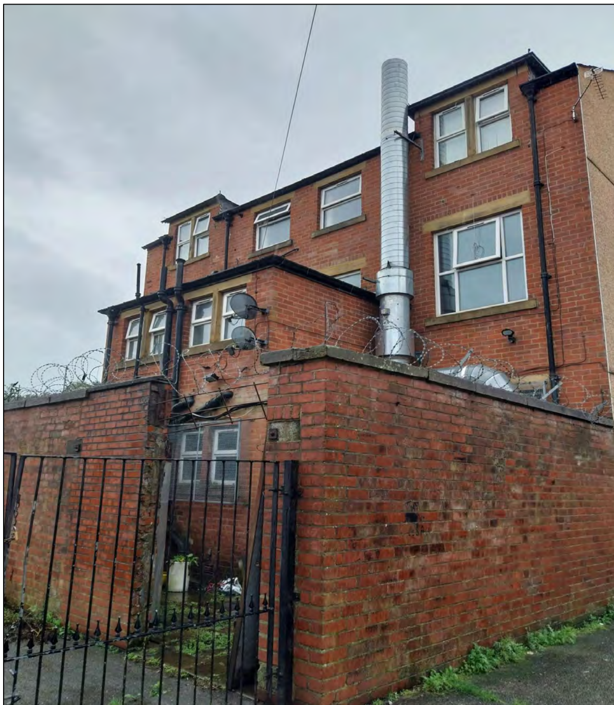
Plate 10 rear view of the properties at 29 to 31 Maclure Road, taken from Fire Station Yard, looking south-west
