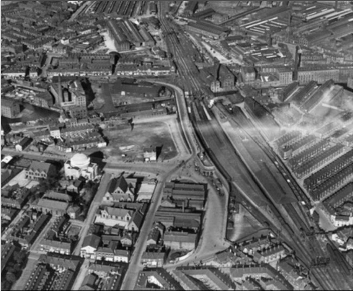
Plate 8 Aerial image showing the Site and surrounding area, taken from Maclure Road Conservation Area Appraisal, courtesy of Britain from above, REF EPW016784
