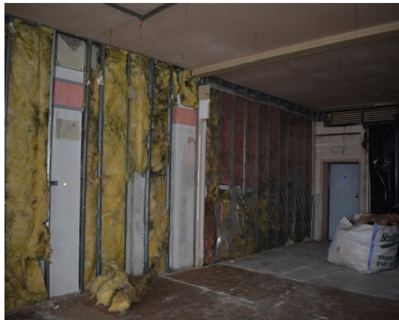
A partial internal strip out of the building has been
