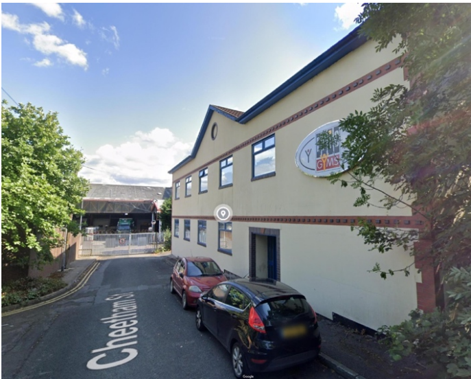
Front Elevation showing existing building materials
