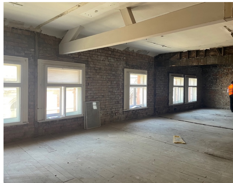
Interior After Strip Out
