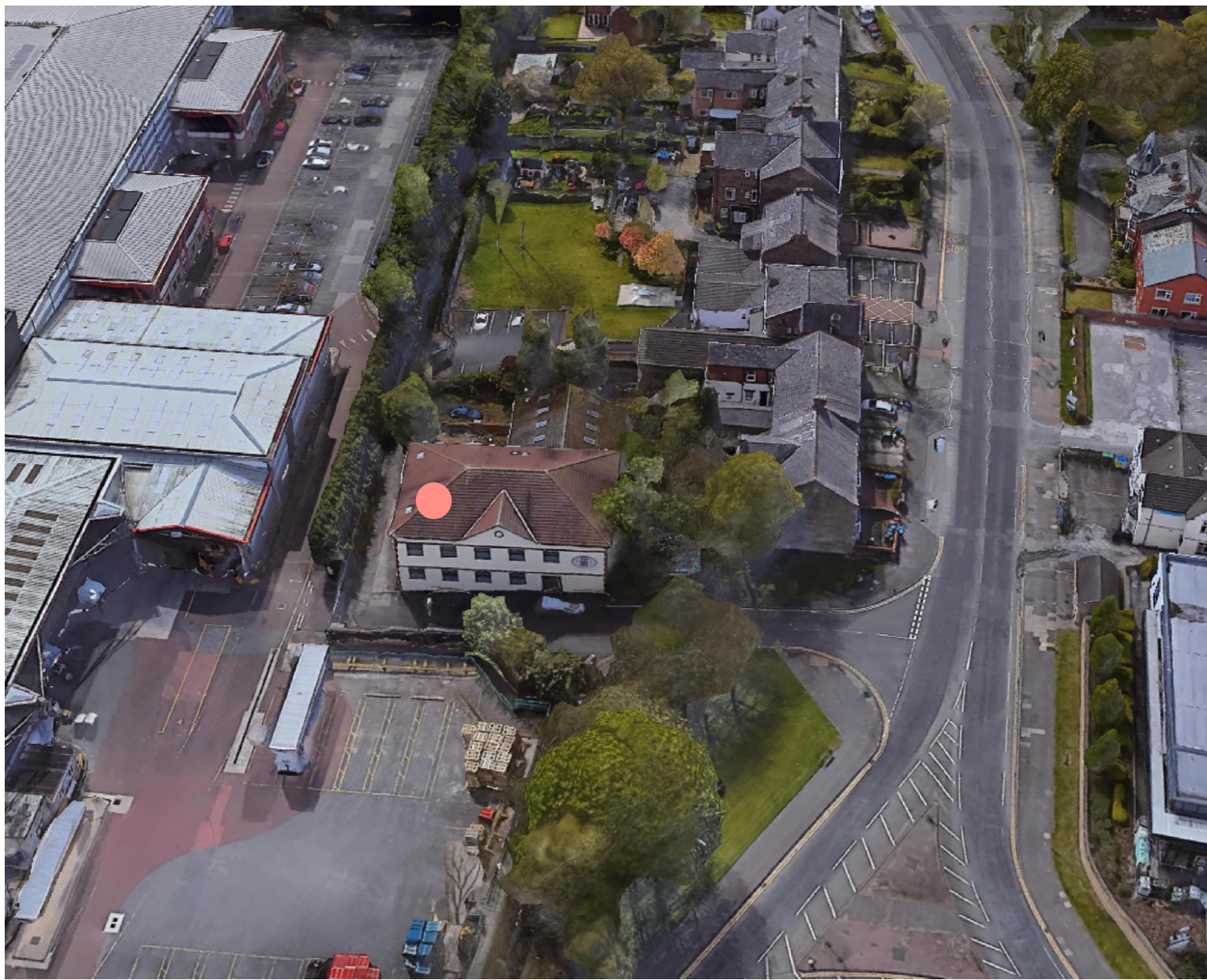
Aerial photograph of the existing building last used as a gym facility
