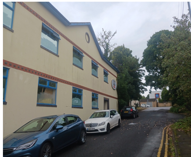
Main façade fronting Cheetham Street
