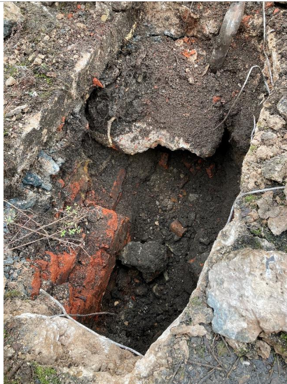
PLATE 4 TP116 EXCAVATION WITH OBSTRUCTIONS
