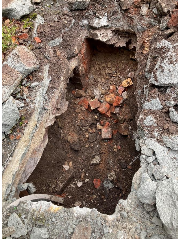
PLATE 5 TP107 EXCAVATION WITH OBSTRUCTIONS
