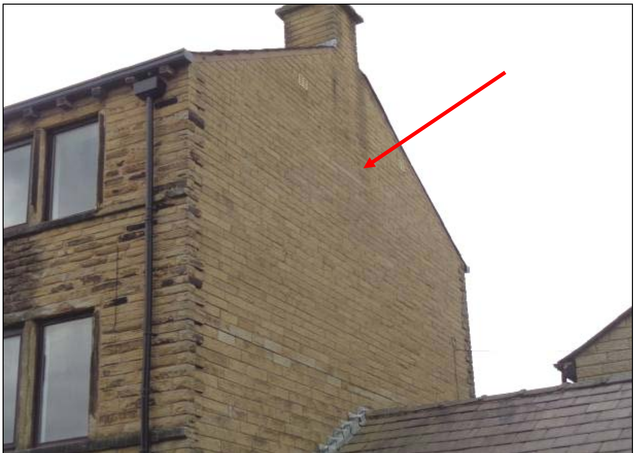
7. The north elevation was rebuilt when the adjoining house was removed
