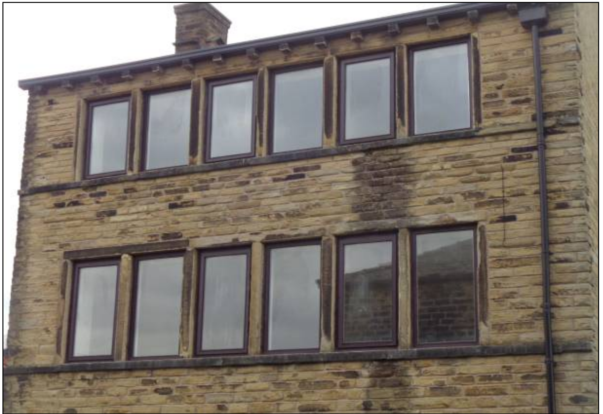
4. Both upper floors were probably used for weaving
