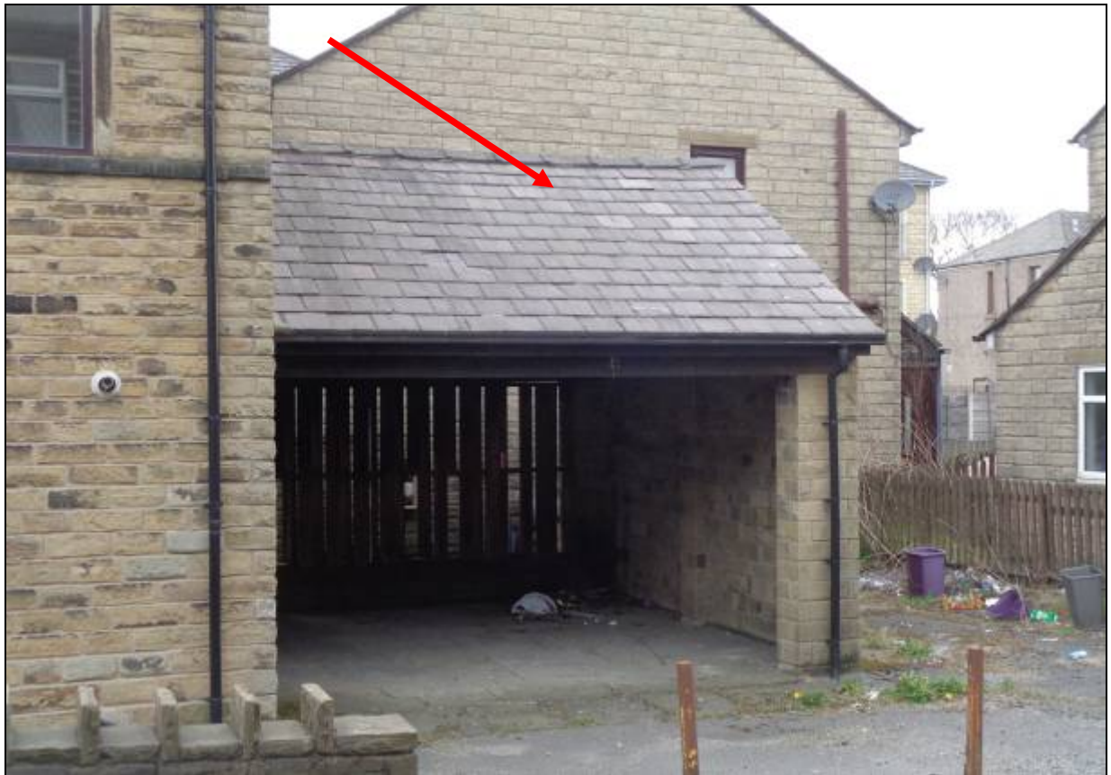
6. Modern car port on north side
