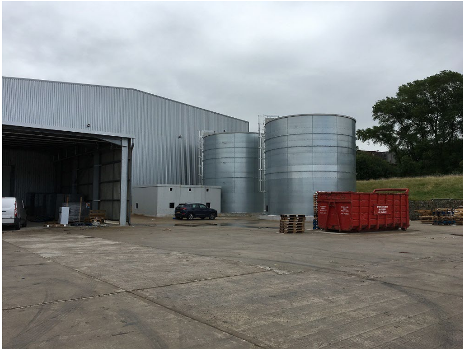
General view from apron
