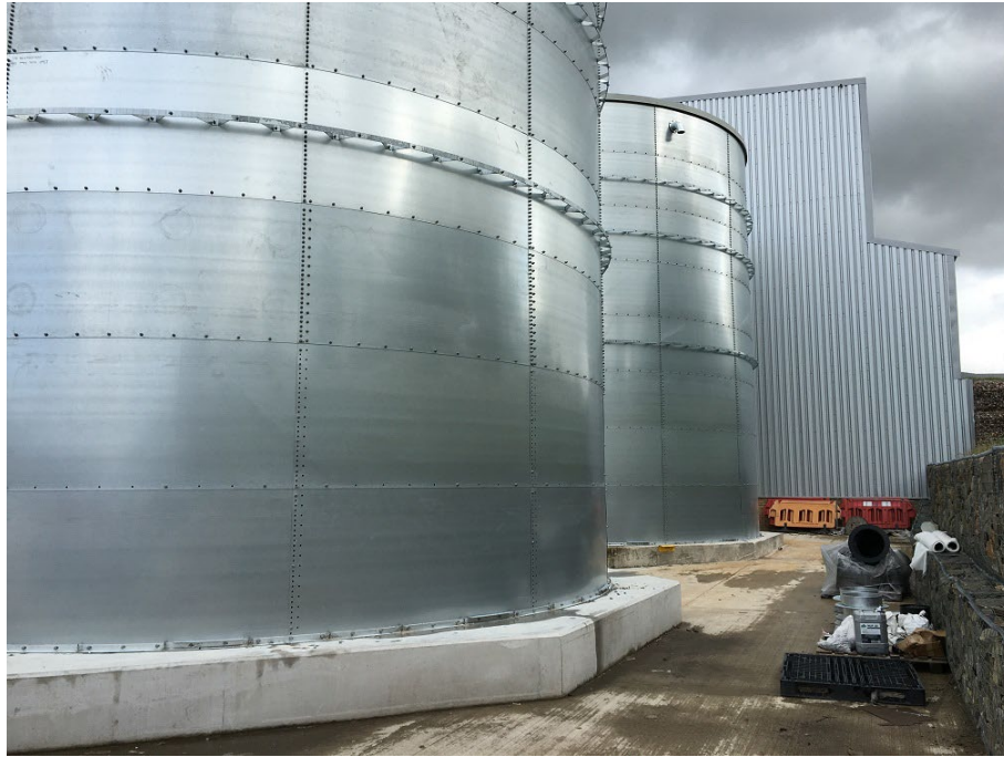
Close up view of tanks from south west
