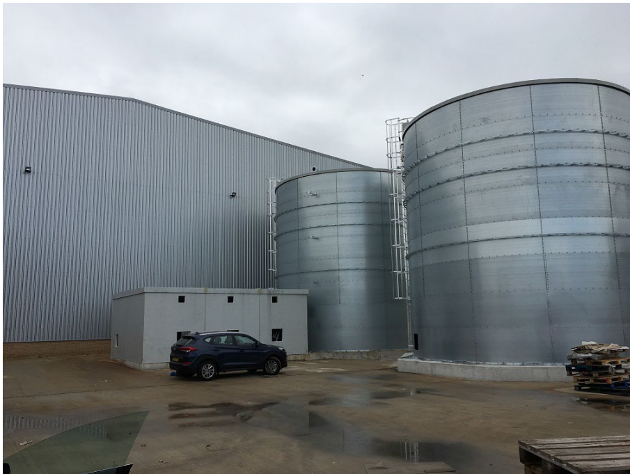
General view from west
