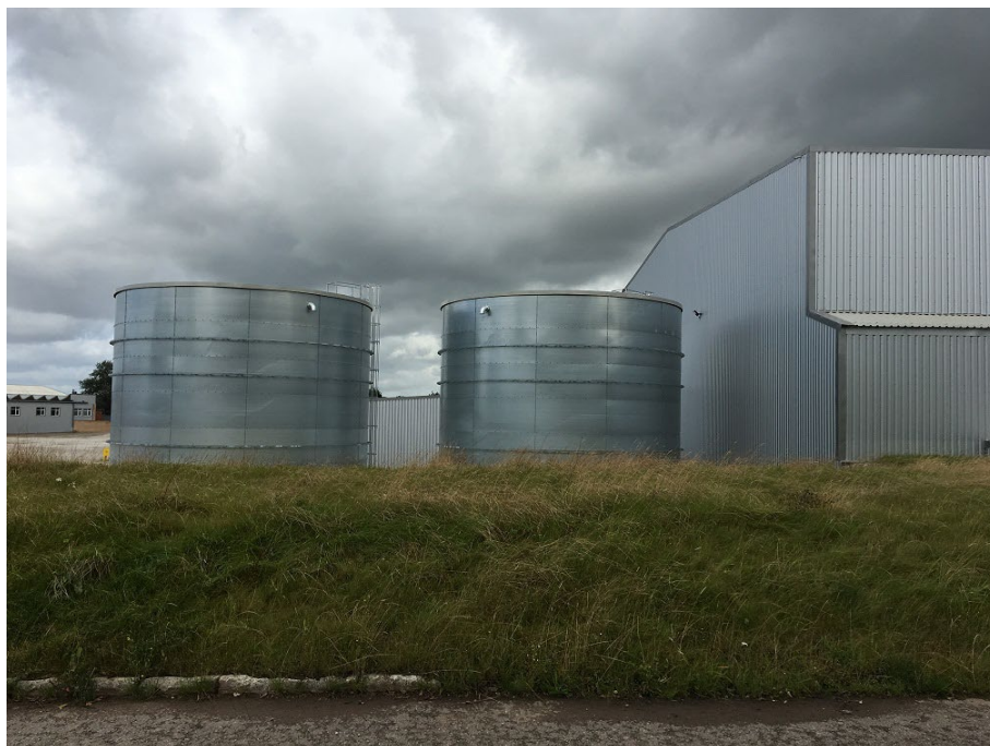
General view of tanks from south east
