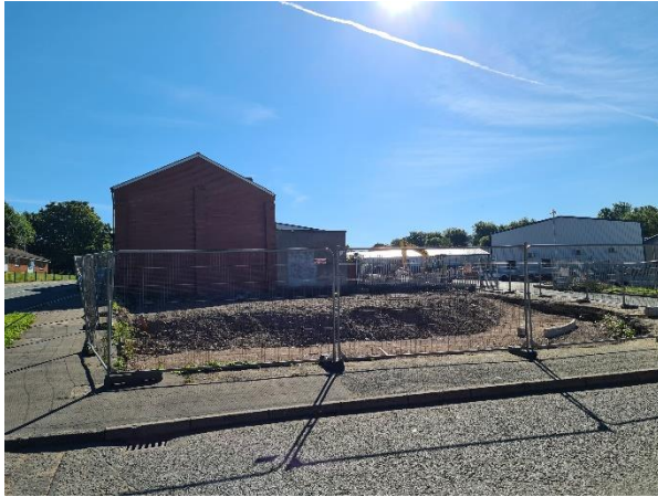
Fig 2.5: View of the site from side road (entrance to industrial estate)
