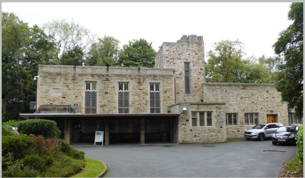
Plate 1. Principal S elevation of Rochdale Crematorium
