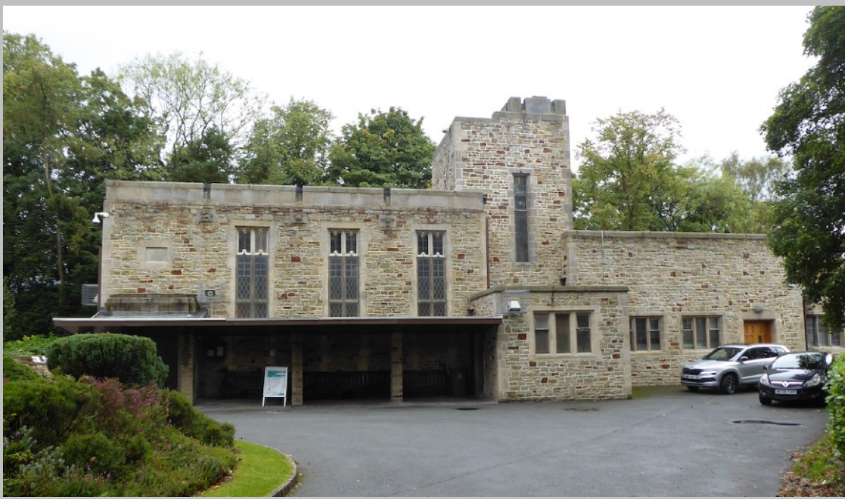
Plate 1. Principal S elevation of Rochdale Crematorium
