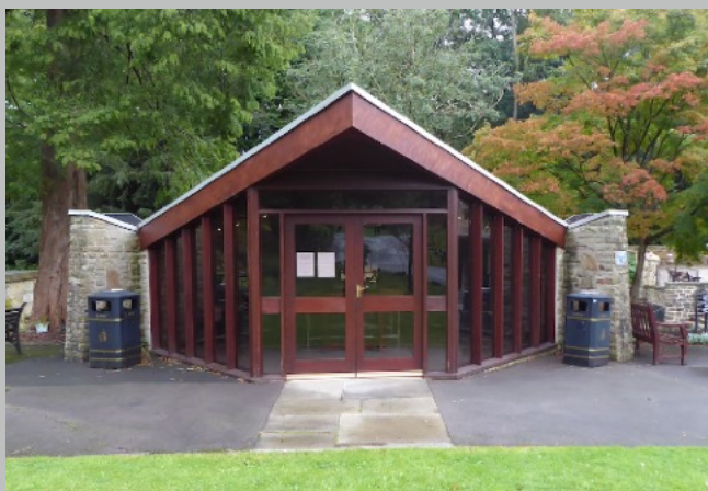
Plate 12. S elevation of Book of Remembrance Building
