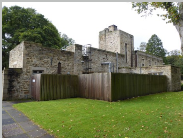
Plate 6. View of rear from NE
